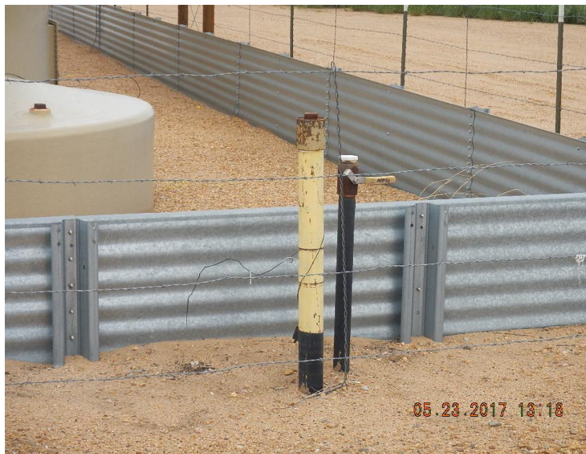
Risers on south side of battery. Not capped or marked. GPS 40.21278, -104.74992
