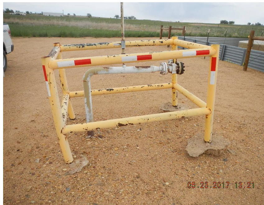
Riser between tank battery and separators Not marked or capped, GPS 40.21337, -104.74999
