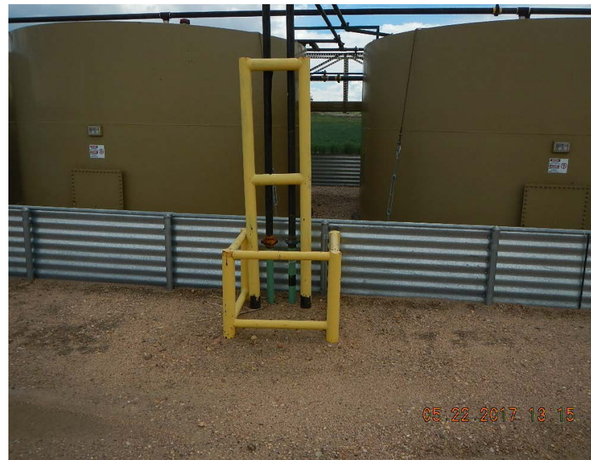
Dump line and vent risers N40.31610 W-104.91039
