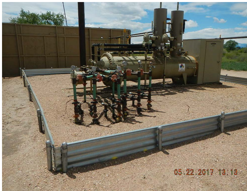
Separator inlet and bypass risers N40.31635 W-104.91036
