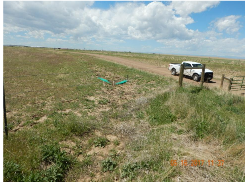
Photo 2. Photo taken from the entrance of location, facing Southwest. Appears a diversion ditch has been installed to control run-on onto location. Wattle BMPs are in need of repair.
