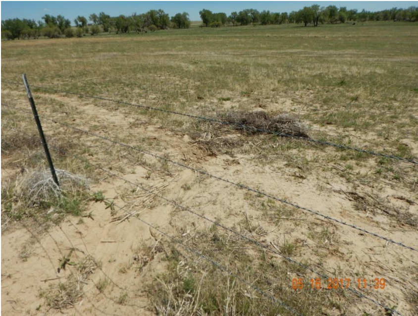
Photo 9. Photo taken along the perimeter of the location and the adjacent land, facing East. The diversion ditch BMP does not have any form of a stabilized outlet structure to prevent sediment laden stormwater from leaving location. It appears sediment is being discharged off location and shall comply under Rule 1002.f.
