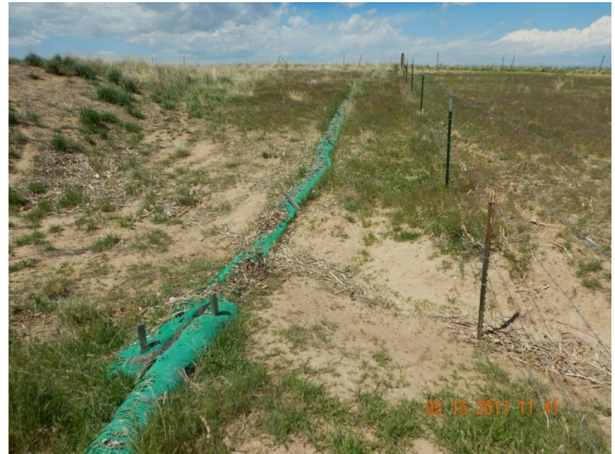
Photo 14. Photo taken along the northwestern perimeter of the location, facing West. Wattle BMPs are in need or repair. It is unclear whether erosion from the oil and gas location has caused a gully formation or whether that was previously existing. Wattle BMPs might be an insufficient BMP by itself to ensure sediment laden stormwater from leaving location.
