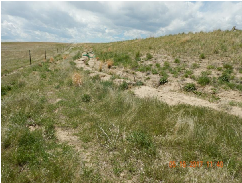
Photo 11. Photo taken along the northeast perimeter of the location, facing South. Diversion ditch BMP installed in conjunction with wattle BMPs which is directed to a sediment trap. Wattle BMPs are in need or repair.
