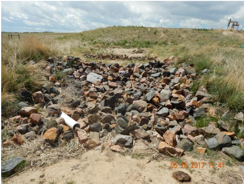
Photo 13. Photo taken along outlet area of the sediment trap, facing South. Outlet protection device BMPs have been installed in conjunction with the sediment trap.
