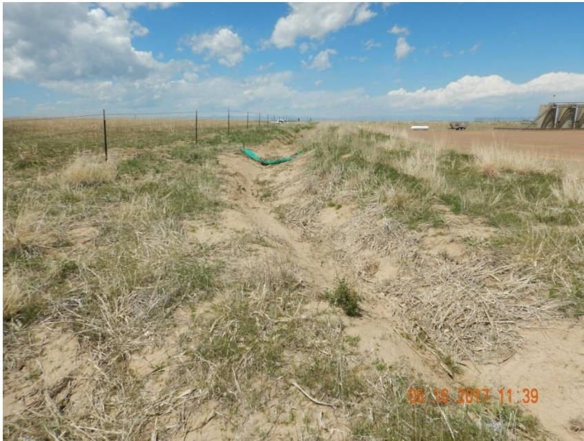
Photo 7. Photo taken from the southeast perimeter of the location, facing West. Photo illustrates the diversion ditch BMP that has been installed to control run-on onto location.
