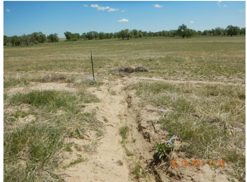
Photo 8. Photo taken from the previous photo location, facing East. The diversion ditch BMP does not have any form of a stabilized outlet structure to prevent sediment laden stormwater from leaving location. It appears sediment is being discharged off location and shall comply under Rule 1002.f.
