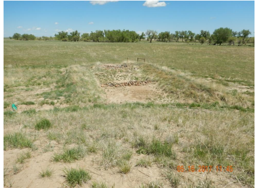
Photo 12. Photo taken from the northeast production area, facing North. Photo illustrates the sediment trap BMP that has been installed.
