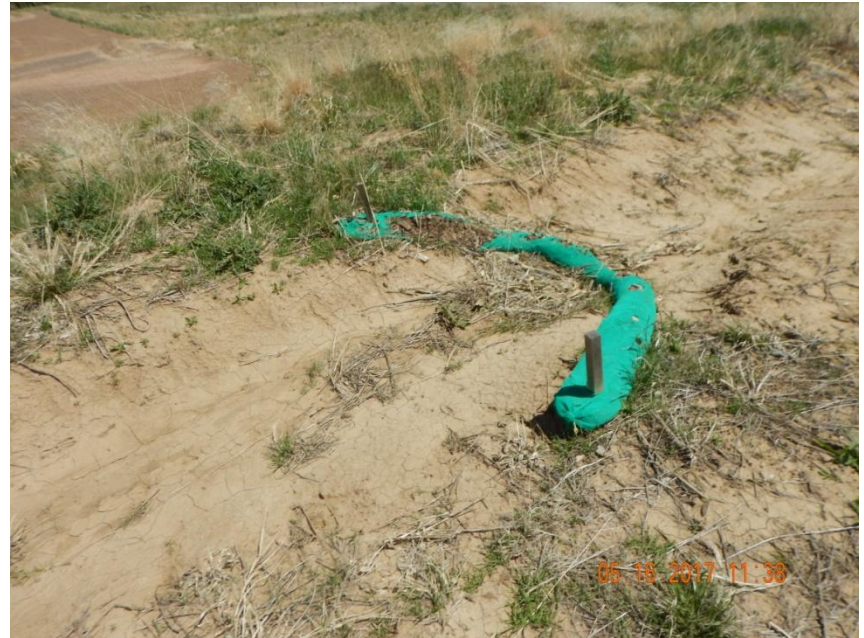
Photo 6. Photo taken along the southern diversion ditch illustrating a wattle BMP in need of repair.
