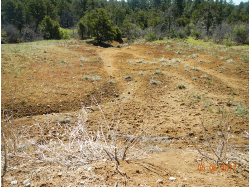
Photo 5: Another view of erosion in the southeastern portion of the project area that needs stabilization.
