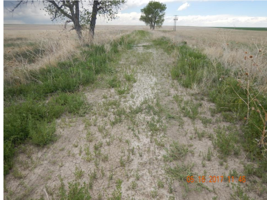
Photo 5: Photo taken from the access road, east of the location facing west. Photo shows access road has not been adequately re-contoured, re-graded and reclaimed.
