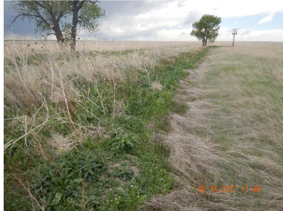
Photo 7: Photo taken from the access road, east of the location facing southwest. Photo shows access road has not been adequately re-contoured, re-graded and reclaimed.
