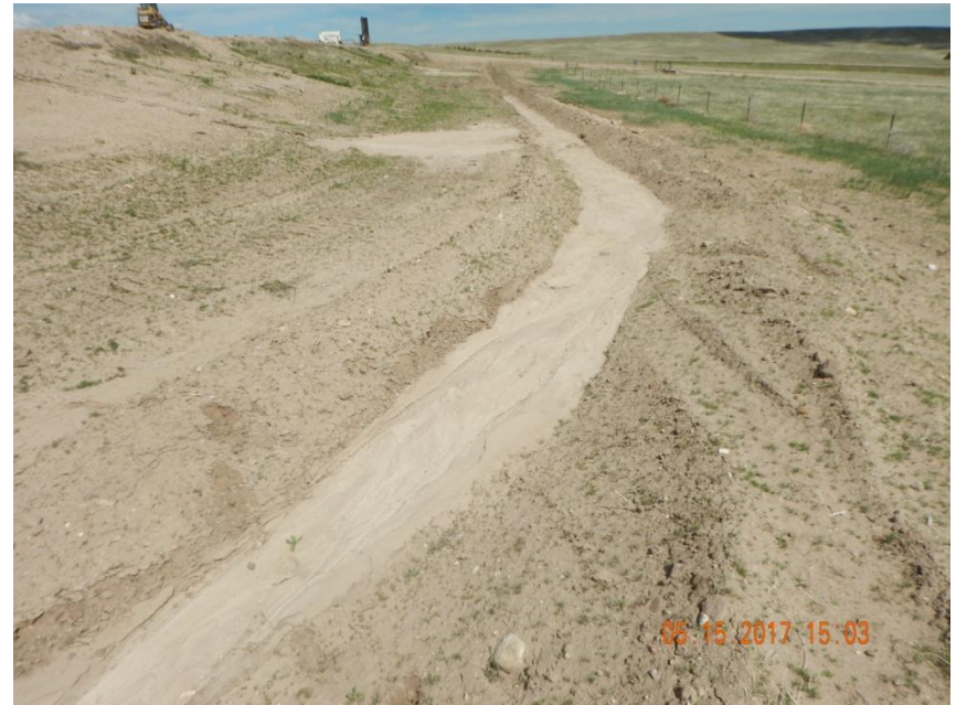
Photo 2. Photo taken from the approximate previous photo location, facing East. Sediment appears to be contained within the stormwater BMP areas of the location.
