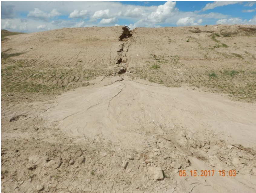
Photo 3. Photo taken of the southwest well pad along the south-facing side, facing North. Gully erosion observed along the well pad perimeter. Sediment appears to be contained within the stormwater BMP areas of the location.
