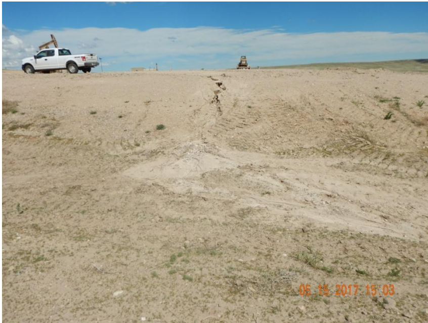
Photo 1. Photo taken of the southwest well pad along the west-facing side, facing East. Gully erosion observed along the well pad perimeter. Sediment appears to be contained within the stormwater BMP areas of the location.
