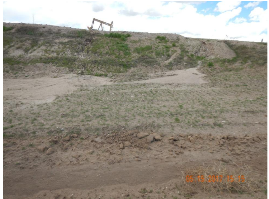
Photo 6. Photo taken along the west entrance of location, facing North. Rill erosion observed along the entrance. Sediment appears to be contained within the stormwater BMP areas of the location.
