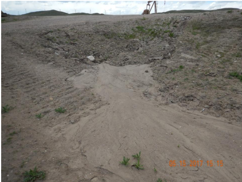
Photo 5. Photo taken along the east entrance of location, facing Northwest. Rill erosion observed along the entrance. Sediment appears to be contained within the stormwater BMP areas of the location.
