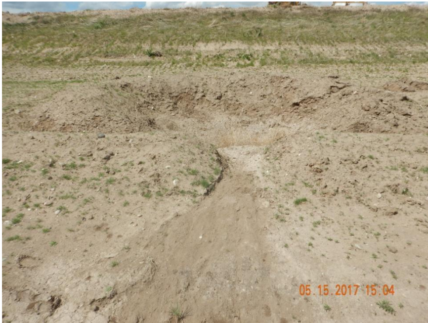
Photo 7. Photo taken from the western sediment trap, facing North. Sediment trap does not have any stabilized outlet protection to prevent sediment laden stormwater from discharging if the sediment trap reaches to capacity.
