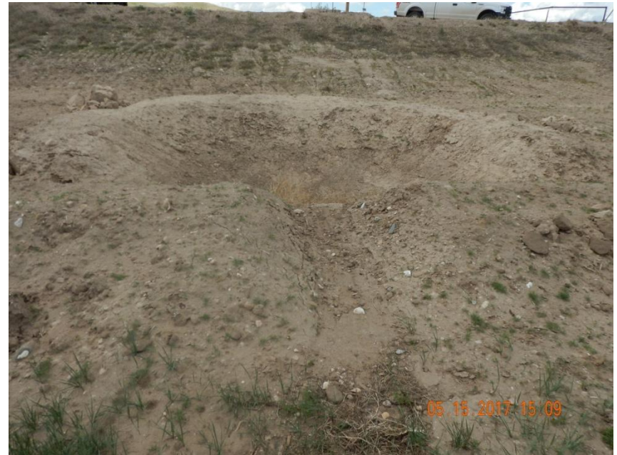
Photo 8. Photo taken from the eastern sediment trap, facing North. Sediment trap does not have any stabilized outlet protection to prevent sediment laden stormwater from discharging if the sediment trap reaches to capacity.
