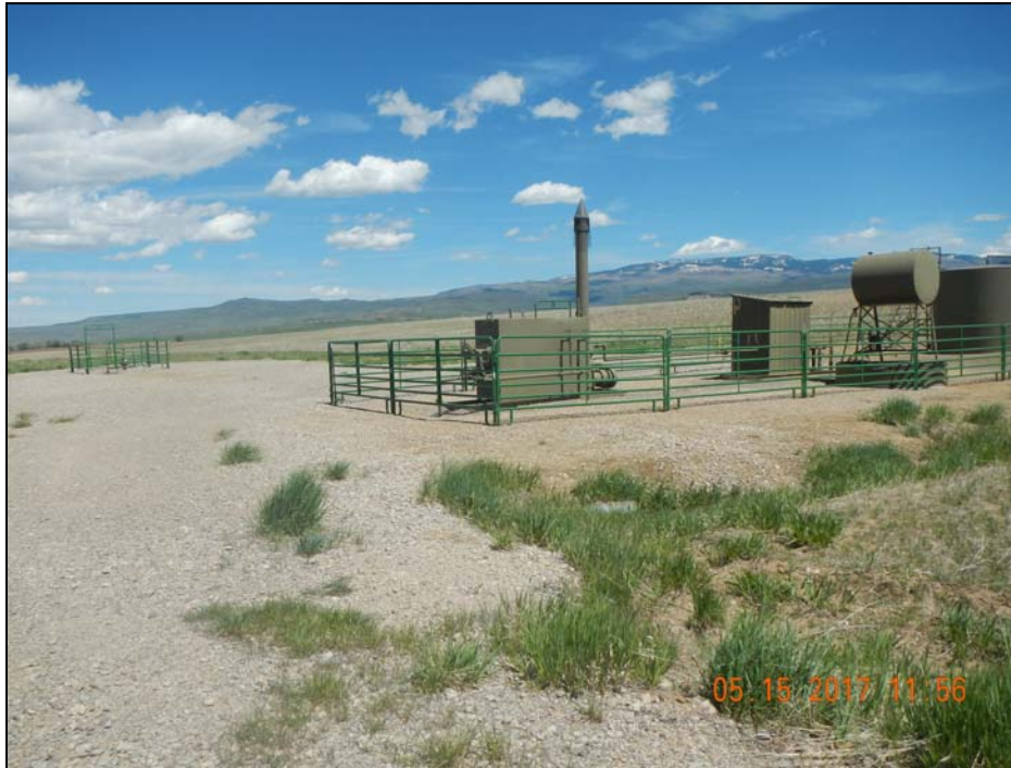
Photo 1. Photo taken at entrance to location facing northwest.
