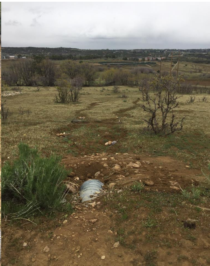
Rill repair around culvert
