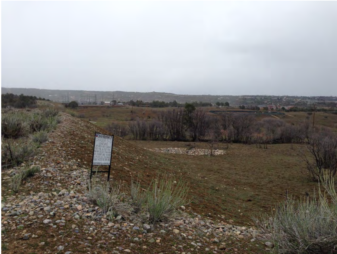
Photo 6 – Crader 3-3 south fill wall and stormwater pond. View to east.
