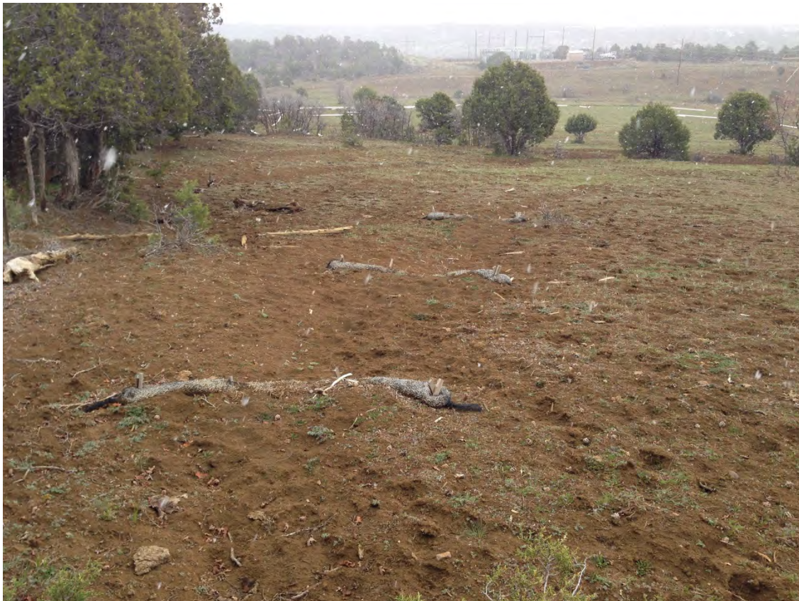
Photo 11 - Upper diversion ditch discharge north end. Note minor rill (to be mitigated). View to east.
