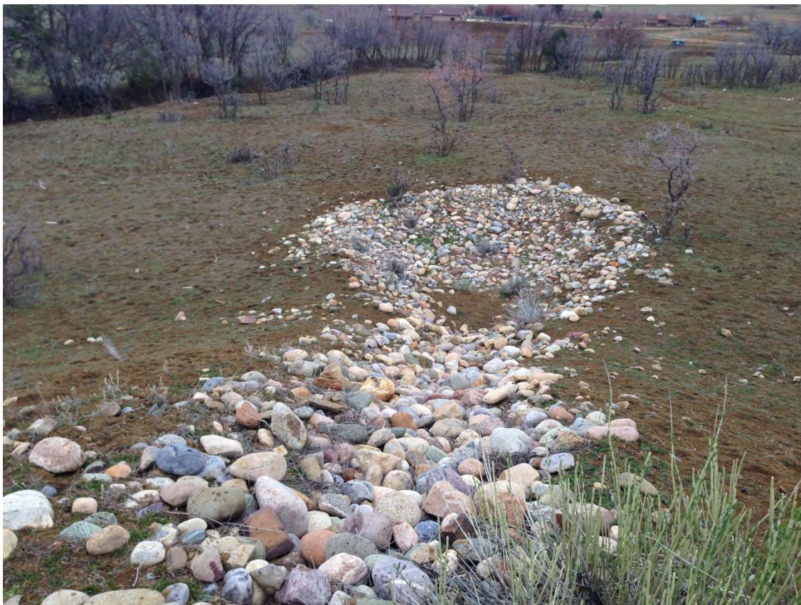
Photo 7 – Crader 3-3 stormwater detention pond. Functional and to remain. View to east.
