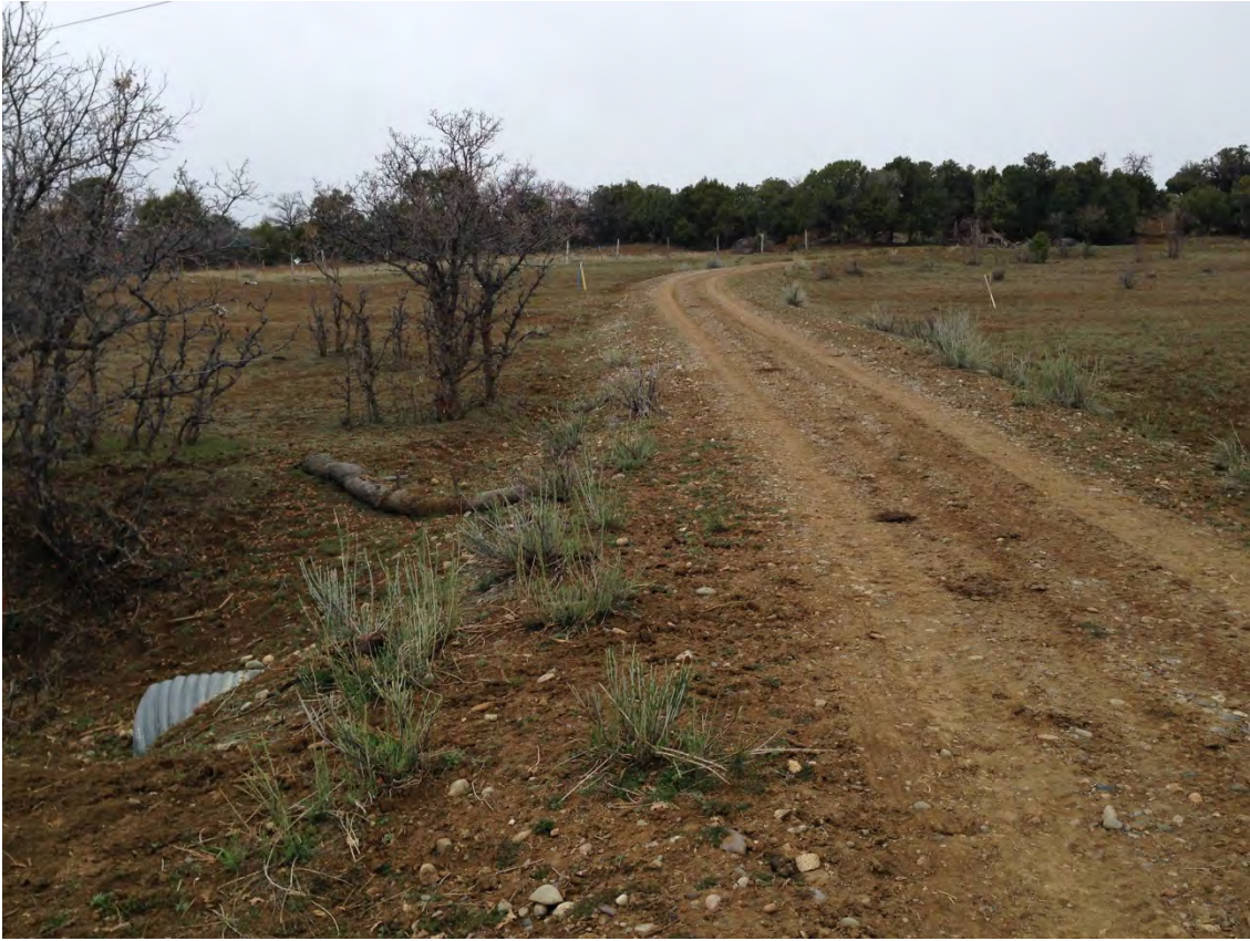
Photo 3 – Crader 3-3 Access Rd crossing irrigation ditch. To remain.
