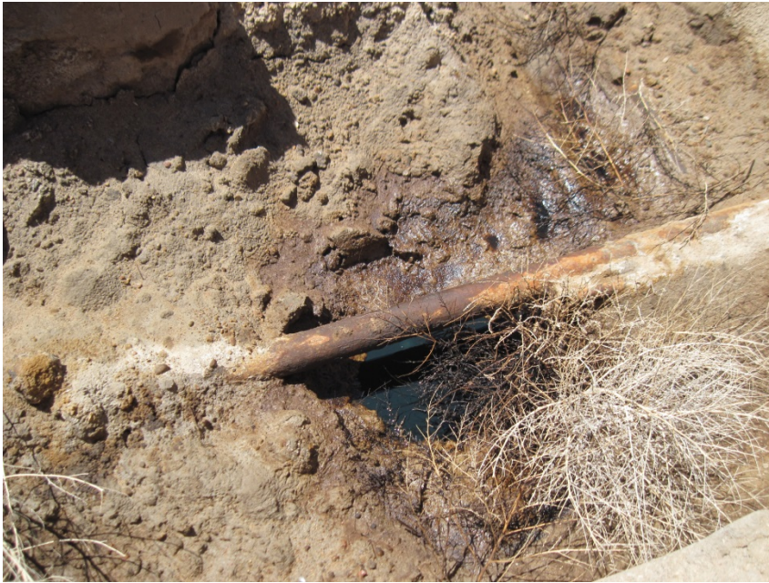
Nels Christian unit #2 Flow line leak
