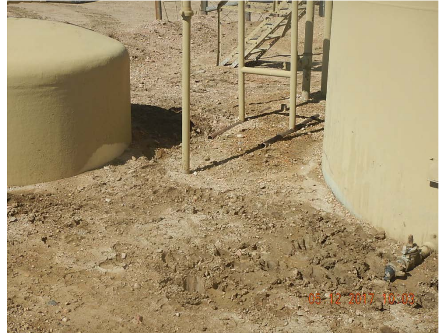
Photo 5: Stained soil removed/remediated
