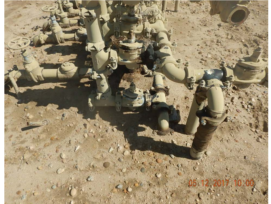
Photo 7: Stained soil at manifold
