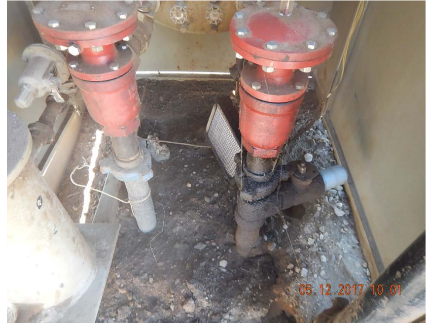
Photo 9: Stained soil removed/remediated
