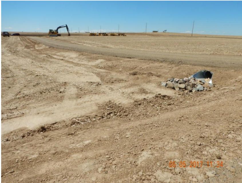
Photo 9. Photo taken from the western access road, facing South. A stabilized outlet has been installed in conjunction with the culvert.
