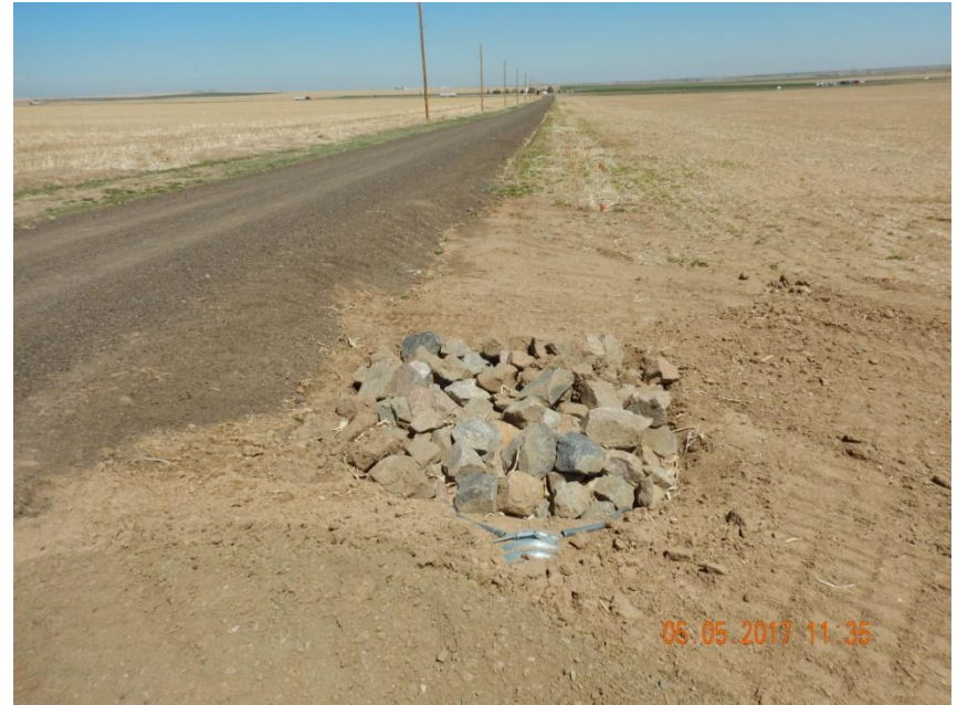
Photo 10. Photo taken from the entrance of location, facing North. A stabilized outlet has been installed in conjunction with the culvert.
