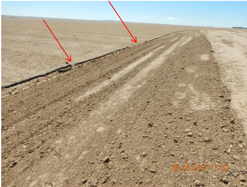
Photo 5. Photo taken from the top of the spoil stockpile, facing South. Filtrexx wattles have been installed around the outer perimeter of the stockpile. Portions of the filtrex are in need of repair/maintenance. Per conversations with the Operator, all stockpiles will be seeded, straw mulched and crimped upon completion of the location.
