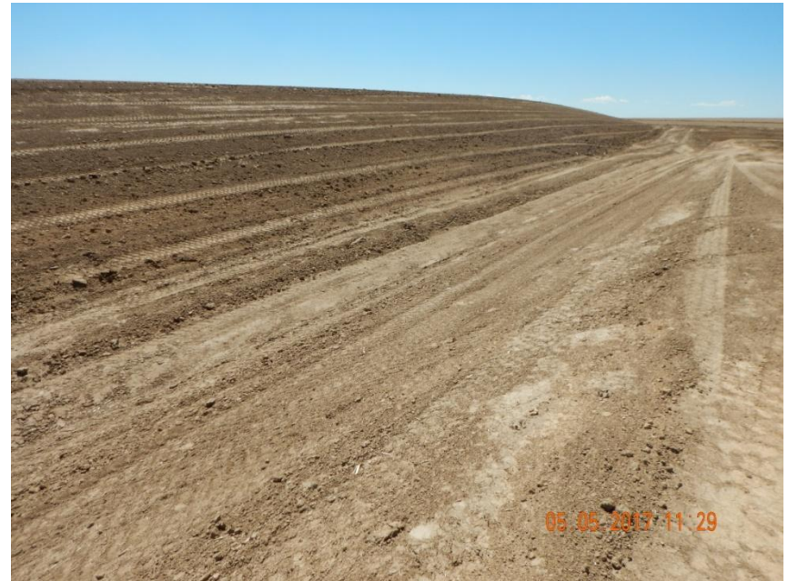
Photo 4. Photo taken from the eastern perimeter of the location, facing Southeast. A spoil stockpile has been stored along the eastern perimeter of the location. Per conversations with the Operator, all stockpiles will be seeded, straw mulched and crimped upon completion of the location.
