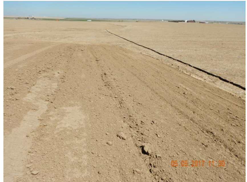
Photo 6. Photo taken from the top of the spoil stockpile, facing North. Filtrexx wattles have been installed around the outer perimeter of the stockpile and portions are in need of repair/maintenance. Per conversations with the Operator, all stockpiles will be seeded, straw mulched and crimped upon completion of the location.
