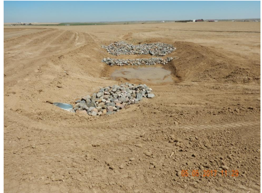
Photo 2. Photo taken from the northeastern location, facing North. Sediment basin has been installed with both inlet and outlet protection devices.
