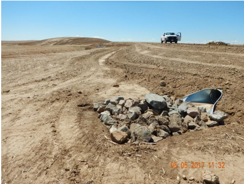
Photo 7. Photo taken from an outlet of a culvert along the east-facing side of the access road, facing South. A stabilized outlet has been installed in conjunction with the culvert.
