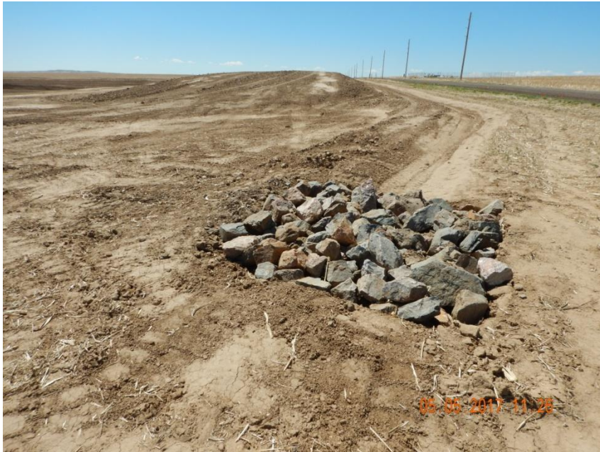
Photo 1. Photo taken north of the topsoil stockpile, facing South. A ditch and berm BMP has been installed around the western location of the stockpile which is directed to a stabilized pit. Per conversations with the Operator, this will be directed to the sediment basin upon completion of the location.
