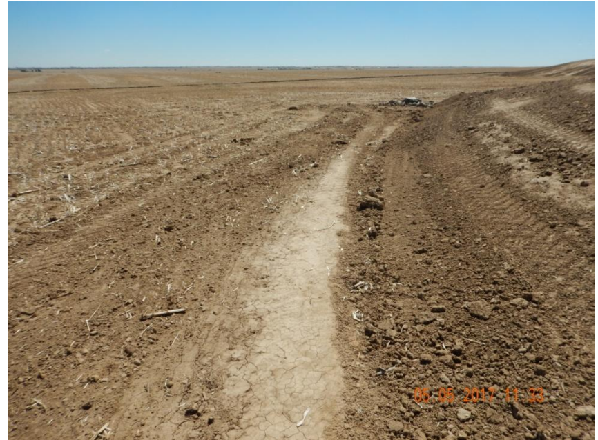
Photo 8. Photo taken along the north-facing side of the same access road in the previous photo, facing East. A shallow ditch has been constructed and appears to be directed to the stabilized outlet used for the culvert.
