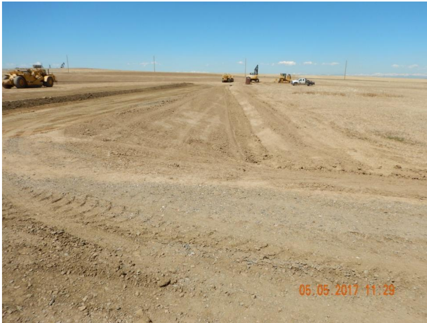
Photo 3. Photo taken from the previous photo location, facing West. A ditch and berm BMP has been installed around the perimeter of the location where stormwater runoff is directed through a culvert to the sediment basin.
