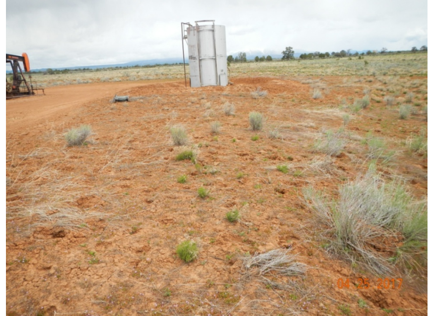
Photo 4: View of the eastern portion of the project area from the southeastern corner facing northward. Two unused ladders are present around the tanks.
