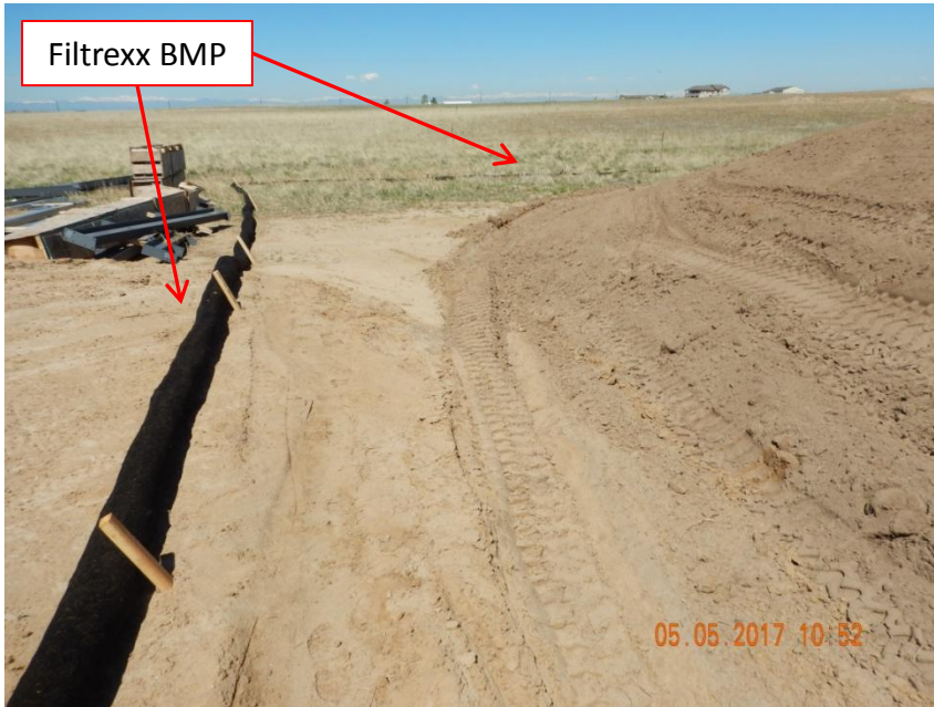
Photo 5. Photo taken from the southwest location, facing West. Temporary stormwater BMP installed around the entire location in the form of a filtrex wattle.
