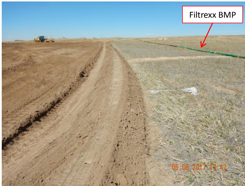
Photo 3. Photo taken from the northeastern location, facing West. Ditch and berm BMP has been installed along the northern perimeter of the well pad location.
