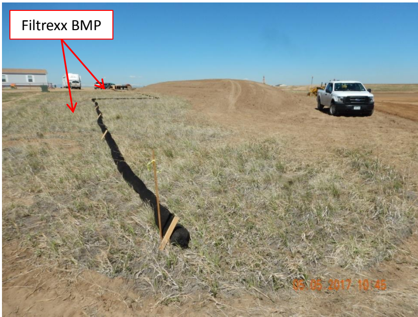
Photo 1. Photo taken from the entrance of location, facing Northwest. Topsoil has been salvaged and stored along the southern perimeter of the location. Temporary stormwater BMP installed around the entire location in the form of a filtrex wattle.
