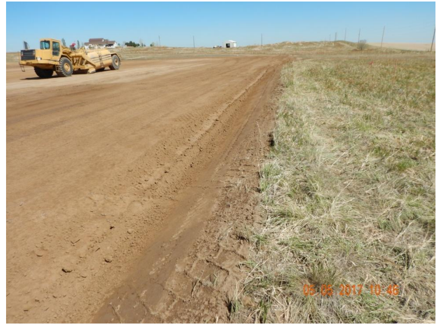
Photo 2. Photo taken from the southeastern location, facing North. Diversion ditch has been installed along the eastern perimeter of the well pad location.
