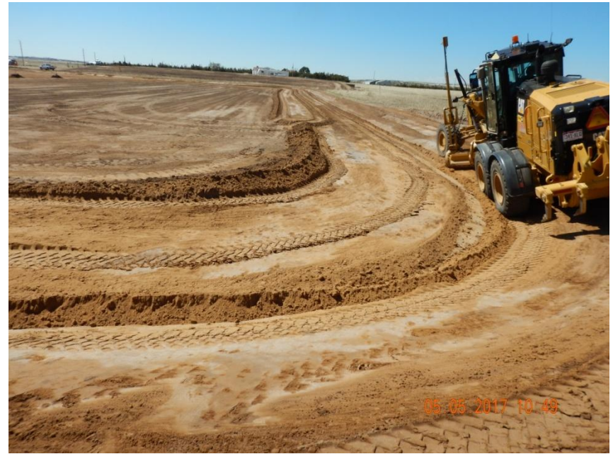
Photo 4. Photo taken from the northwestern location, facing South. Operator is making another pass along the western cut slope.
