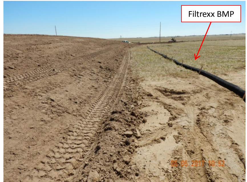
Photo 6. Photo taken from the southwest location, facing East. Temporary stormwater BMP installed around the entire location in the form of a filtrex wattle.
