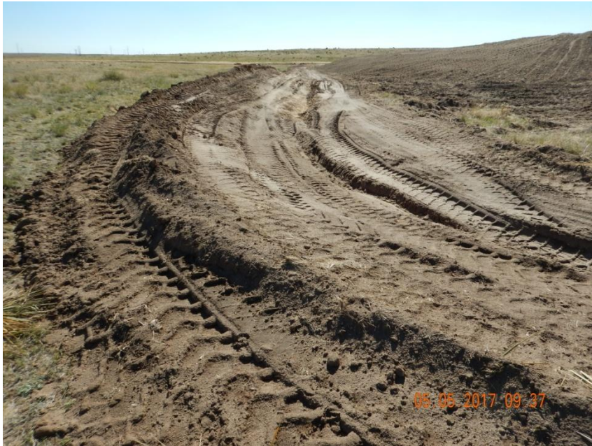
Photo 7. Photo taken from the northwest location, facing East. Berm BMP material does not appear to be sufficiently compacted to ensure unconsolidated soil material does not discharge from location.
