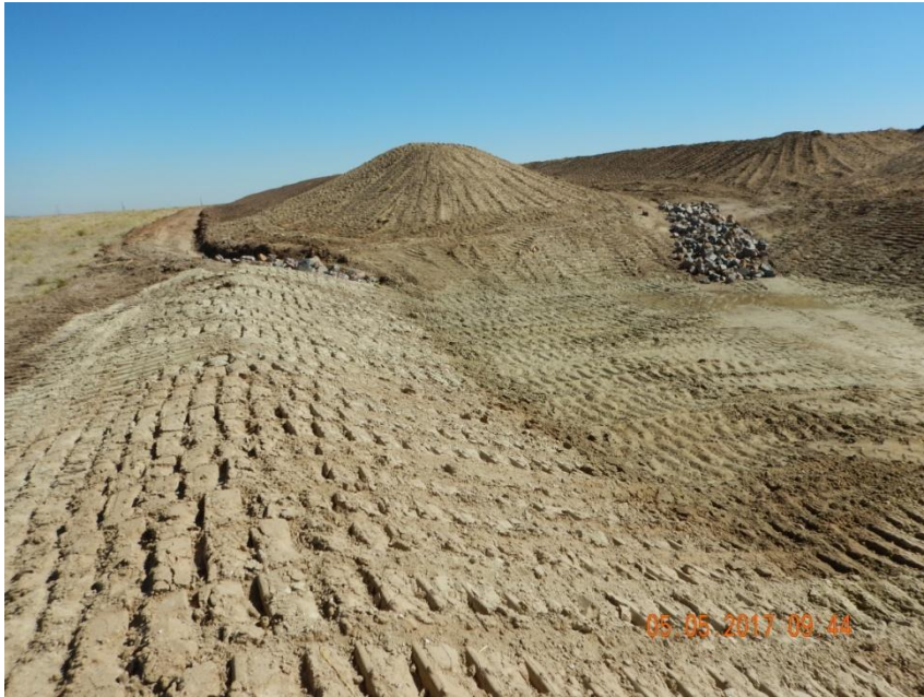
Photo 11. Photo taken from the western sediment basin, facing North. All slopes have been tracked up and down to reduce runoff erosion potential. Photo illustrates inlet protection to the sediment basin.
