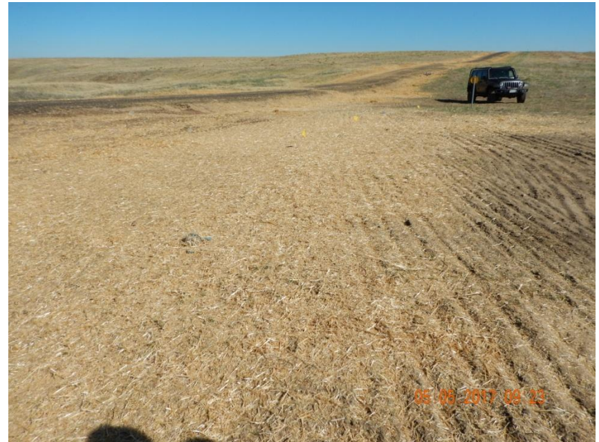
Photo 2. Photo taken from the previous photo location, facing North. All disturbance areas will be seeded, straw mulched and crimped.
