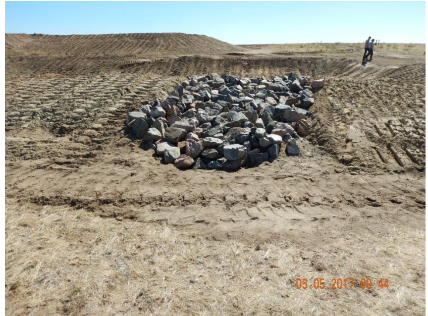
Photo 12. Photo taken from the western sediment basin, facing South. Photo illustrates outlet protection for the sediment basin.
