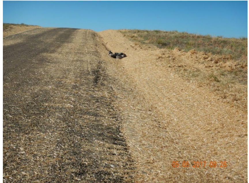
Photo 4. Photo taken from the approximate previous photo location, facing South. All disturbance areas will be seeded, straw mulched and crimped. Check dam material has been placed along portions of the ditch and will be installed so that it is not just a pile of rocks.
