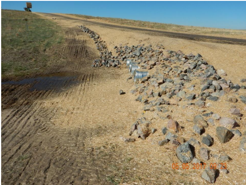
Photo 1. Photo taken along a drainage area on the east side, facing South. Rip rap has been installed around the fill slopes of the culverts; rip rap has been installed along the ditch area leading to the drainage area; road ditch areas have been seeded and mulching IN-PROCESS.
