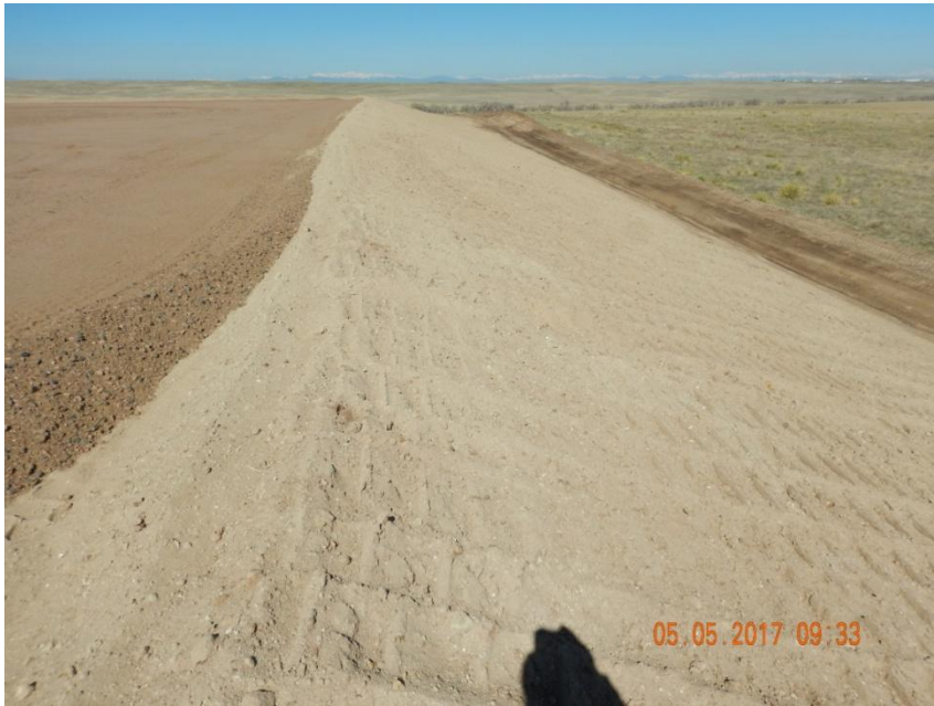
Photo 5. Photo taken from the northern fill slope, facing West. Photo illustrates tracking with equipment up and down the slope to reduce runoff erosion potential.
