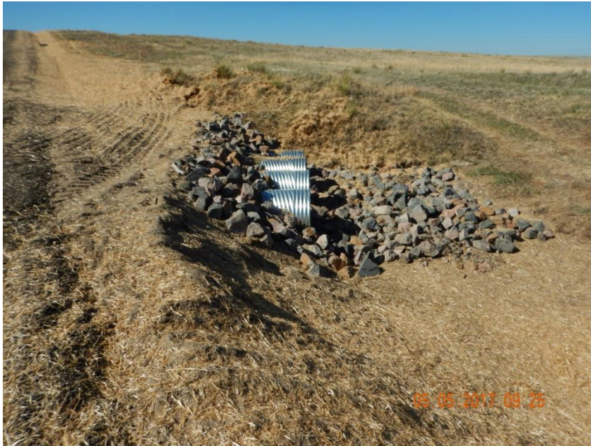
Photo 3. Photo taken along a drainage area on the west side, facing South. Rip rap has been installed around the fill slopes of the culverts; rip rap has been installed along the outlet area; road ditch areas have been seeded and mulching IN-PROCESS.
