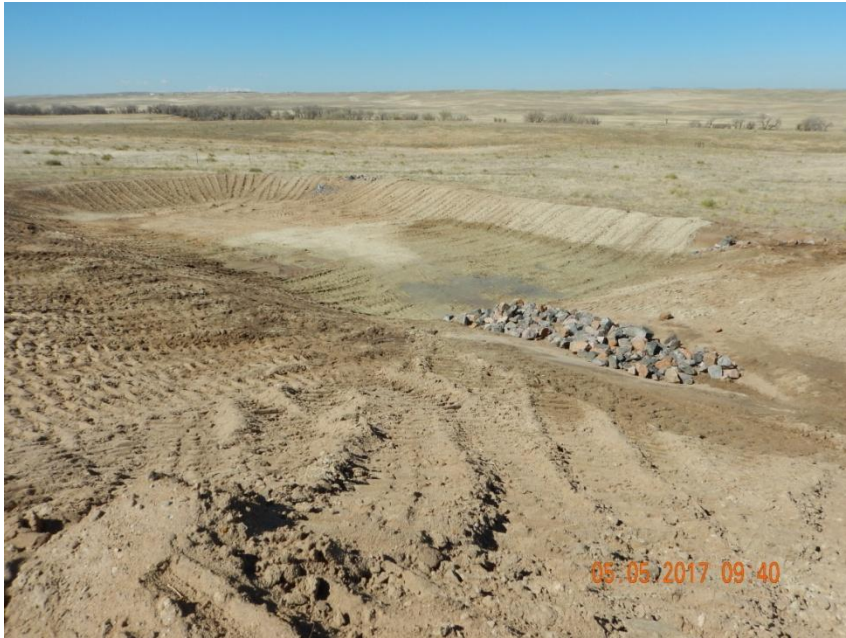
Photo 9. Photo taken from the southwest perimeter of the location, facing Southwest. A sediment basin has been installed in conjunction with inlet and outlet protection devices.
