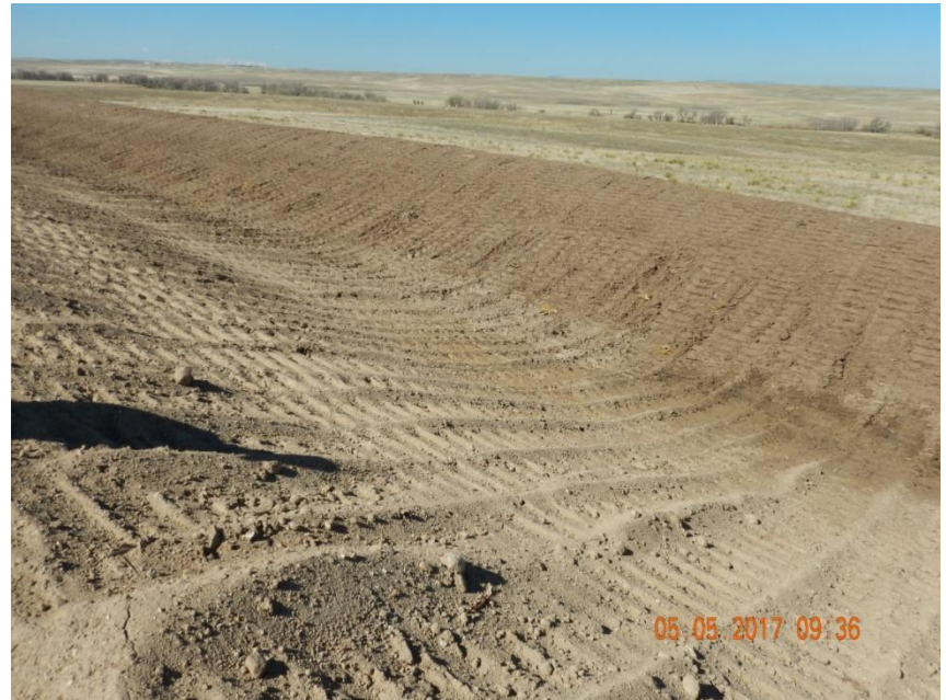
Photo 6. Photo taken from the western fill slope and topsoil stockpile, facing Southwest. Photo illustrates tracking with equipment up and down the slope to reduce runoff erosion potential.
