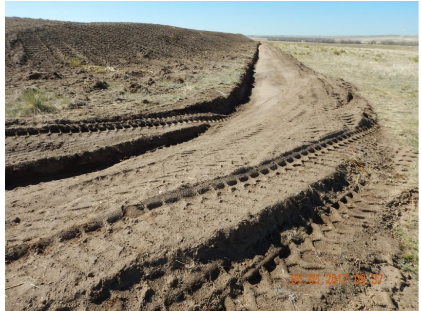
Photo 8. Photo taken from the northwest location, facing South. Berm BMP material does not appear to be sufficiently compacted to ensure unconsolidated soil material does not discharge from location.
