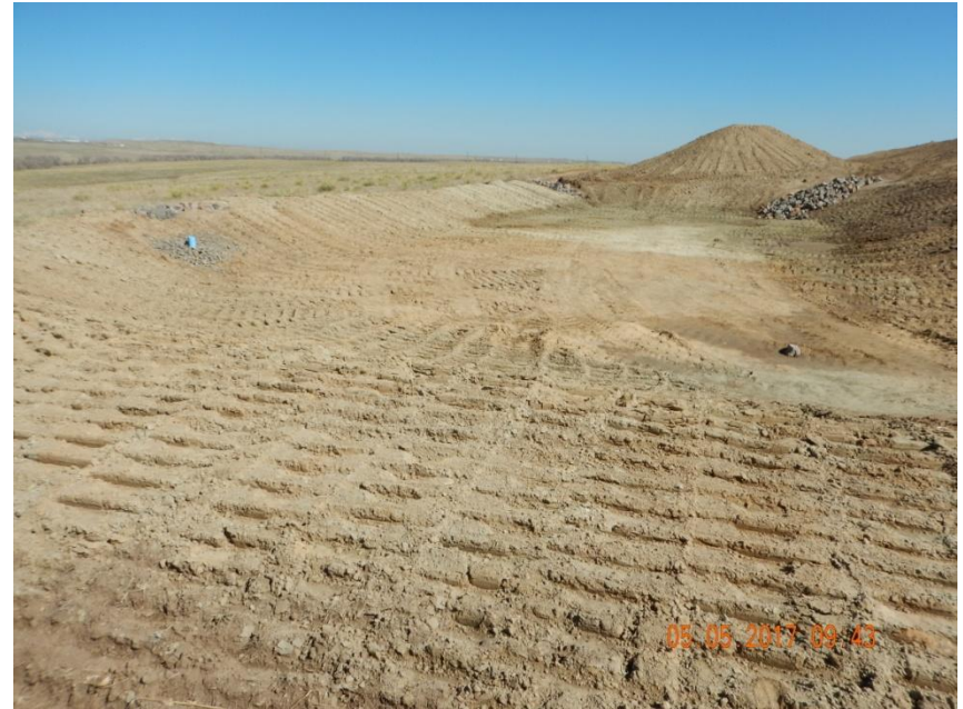
Photo 10. Photo taken from the southern sediment basin, facing North. All slopes have been tracked up and down to reduce runoff erosion potential.
