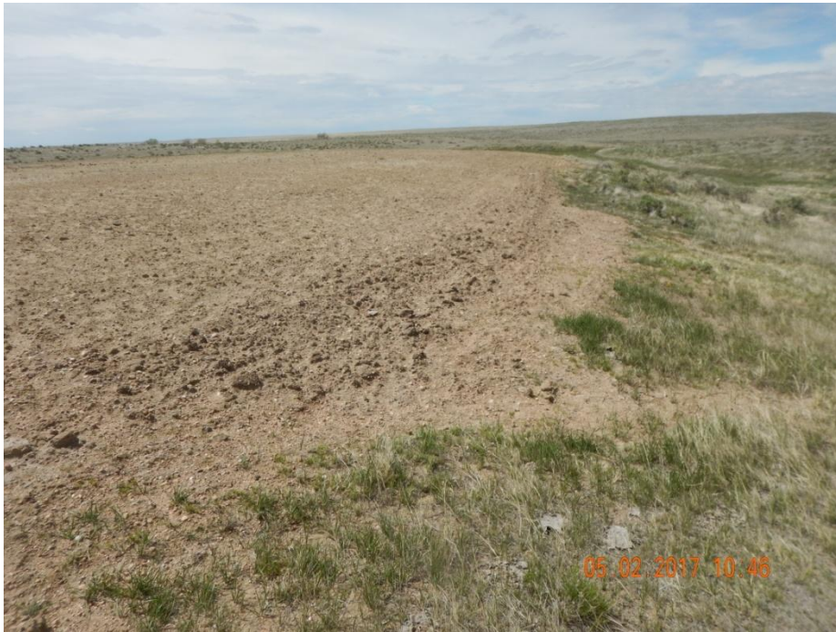
Photo 11: Photo taken from the northwest corner of the pad, facing south. Photo shows areas of the pad that previous inspections had identified erosion concerns. Photo shows erosion has been repaired, however, it does not appear that BMPs have been implemented per the CA. Area appears to be stabilized at time of inspection; continue to perform stormwater management and maintenance until final reclamation passes.
