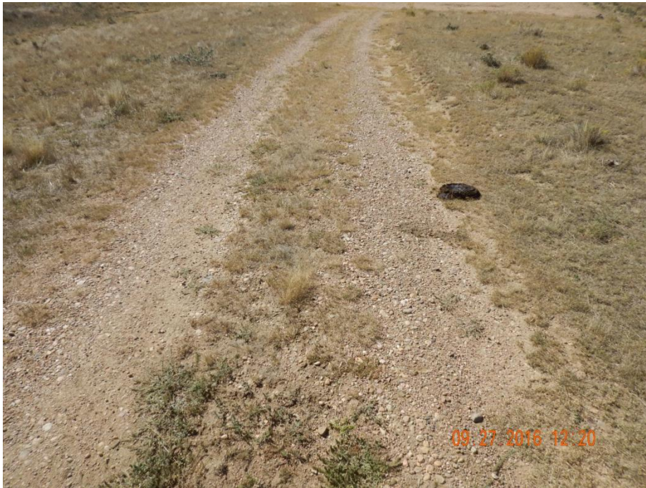
Photo 3: Photo from previous inspection dates 9/27/2016. Photo shows ruts and gravel of access road.
