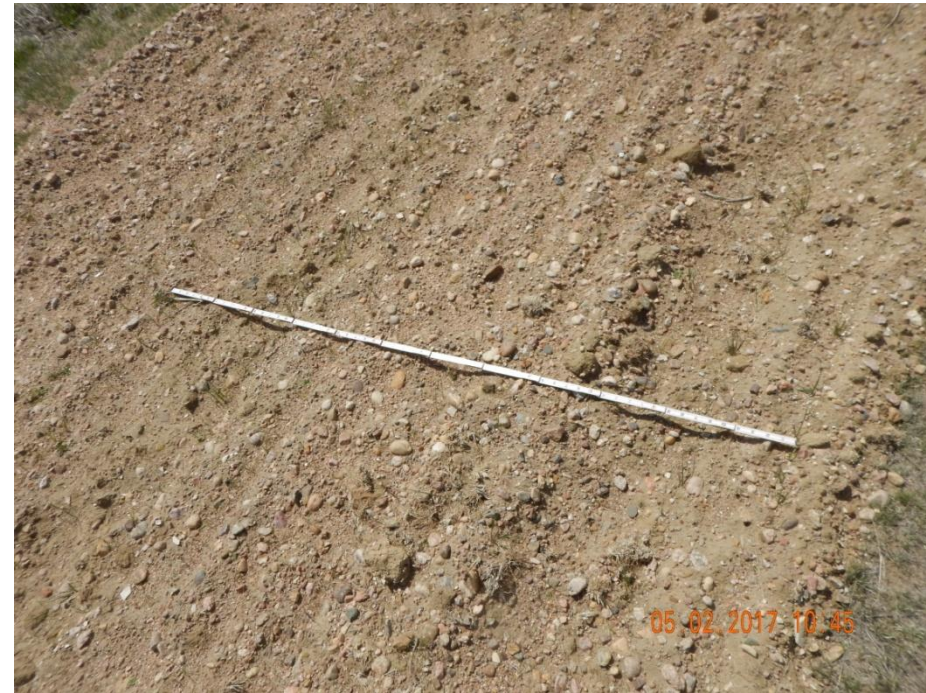
Photo 4: Photo taken from access road, west of the location. Photo shows that though it appears access road had been reseeded, gravel has not been removed per corrective actions from inspection doc. #682501380. 6 foot measuring stick for reference.
