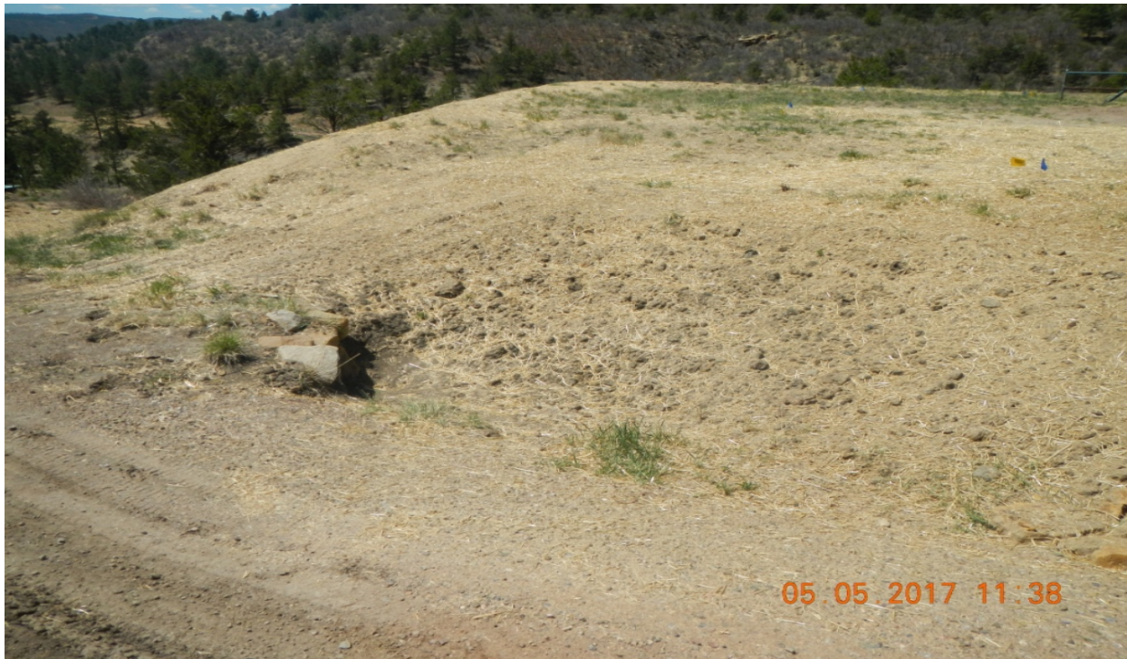
photo 3: The culvert at the location has been maintained and areas of the pad were seeded and mulched.
