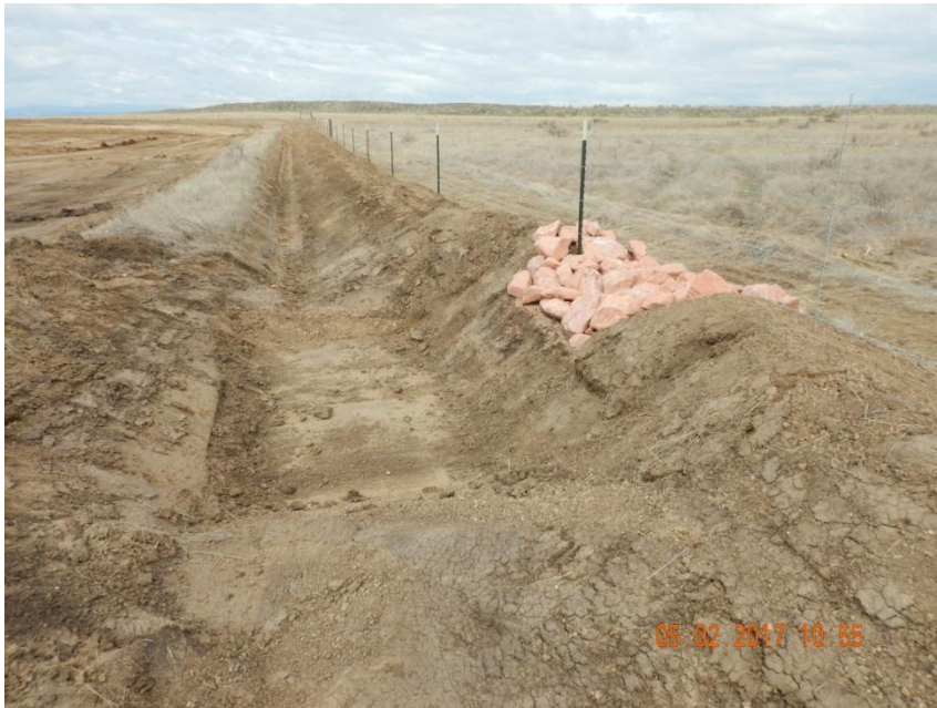
Photo 3. Photo taken from the northeastern location, facing South. Sediment trap has been installed and appears to be in the completion process.
