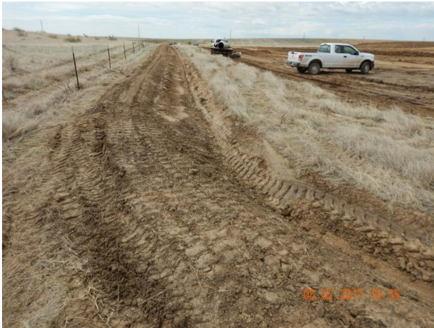
Photo 1. Photo taken from the northeast perimeter of the location, facing South. Ditch and berm BMP has been installed around the entire perimeter of the location.
