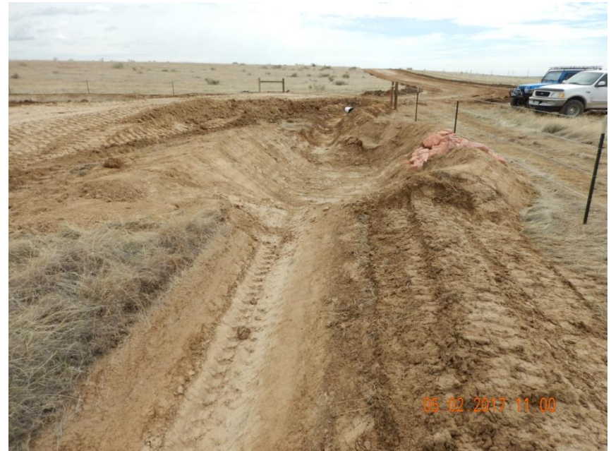
Photo 8. Photo taken from the entrance of location, facing East. Sediment trap has been installed and appears to be in the completion process.
