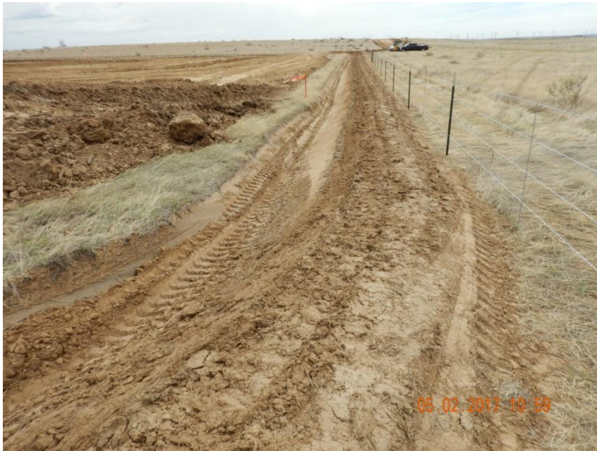
Photo 7. Photo taken from the southwest perimeter of the location, facing East. Ditch and berm BMP has been installed around the entire perimeter of the location.
