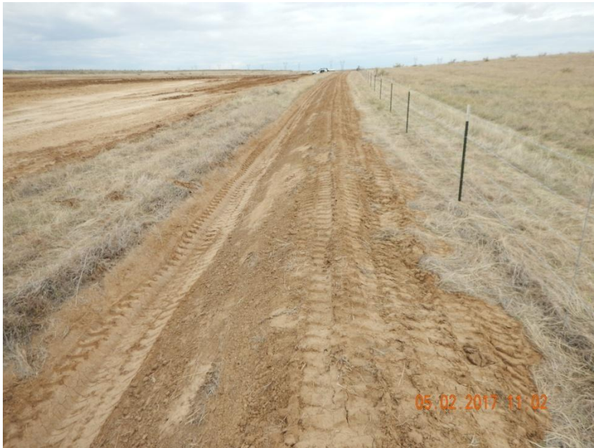
Photo 11. Photo taken from the southeast perimeter of the location, facing North. Ditch and berm BMP has been installed around the entire perimeter of the location.
