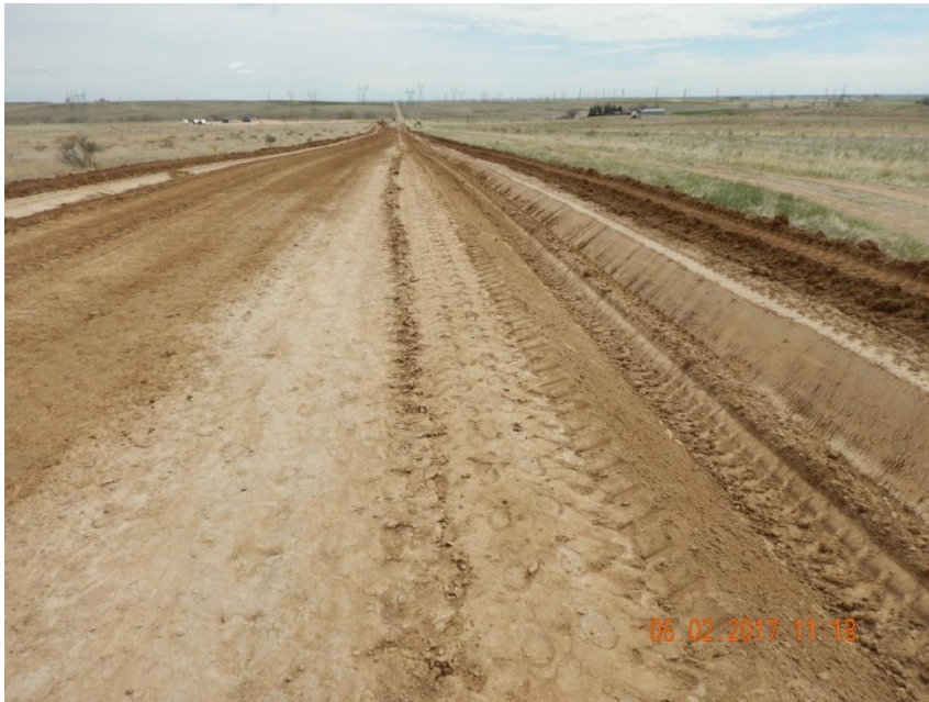
Photo 13. Photo taken from the south side along a portion of the access road, facing East. Diversion ditch has been installed along both sides of the access road.
