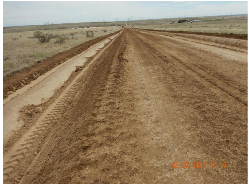
Photo 12. Photo taken from the north side along a portion of the access road, facing East. Diversion ditch has been installed along both sides of the access road.
