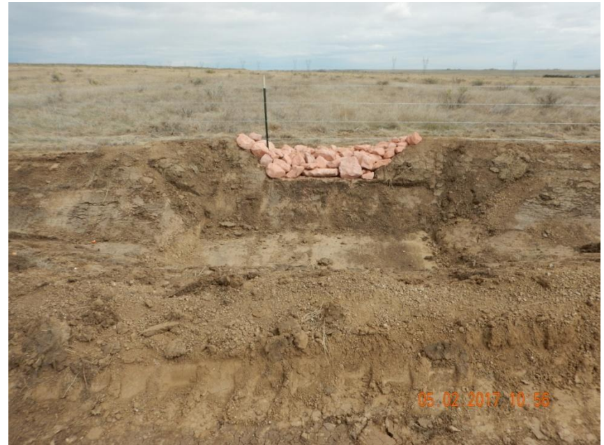
Photo 4. Photo taken from the sediment trap, facing North. Stabilized outlet protection has been installed.
