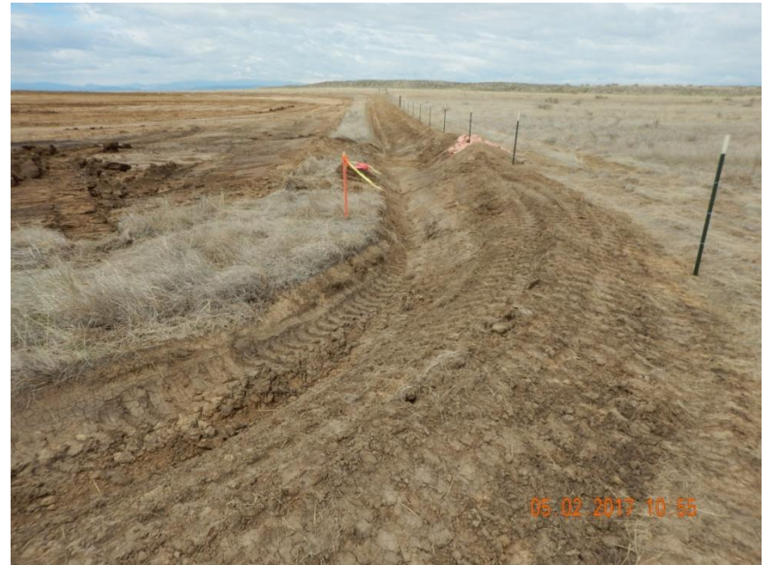
Photo 2. Photo taken from the northeast perimeter of the location, facing West. Ditch and berm BMP has been installed around the entire perimeter of the location.
