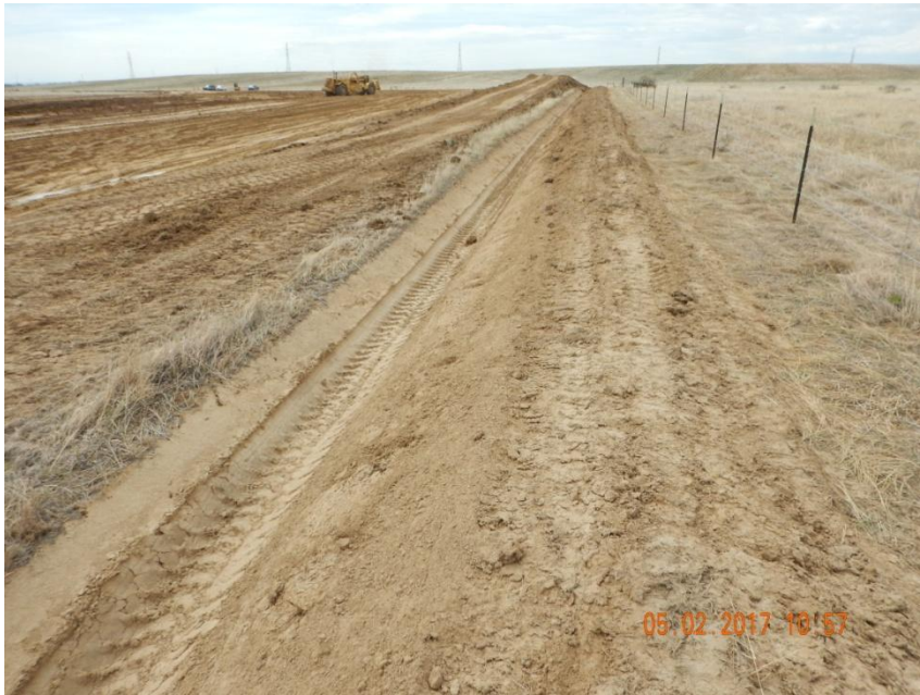
Photo 5. Photo taken from the northwest perimeter of the location, facing South. Ditch and berm BMP has been installed around the entire perimeter of the location.
