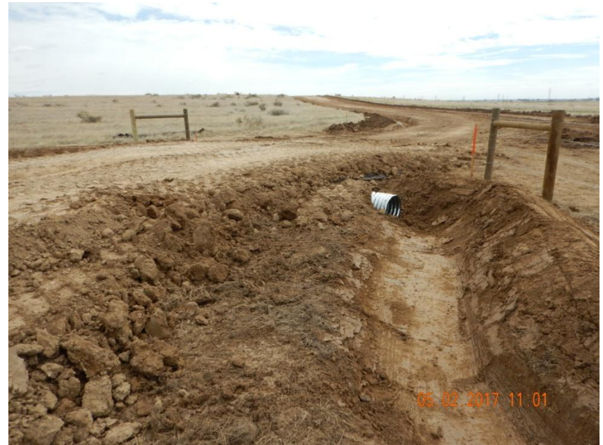
Photo 10. Photo taken from the entrance of location, facing East. Culvert has been installed in conjunction with the ditch and berm BMP.
