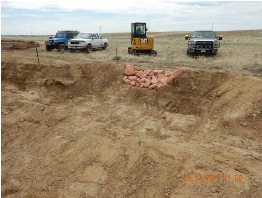
Photo 9. Photo taken from the sediment trap, facing South. Stabilized outlet protection has been installed.
