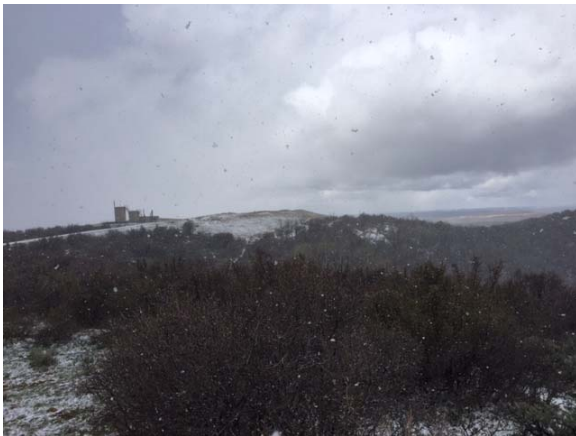
PAD OVERALL LOOKING NORTHERLY
