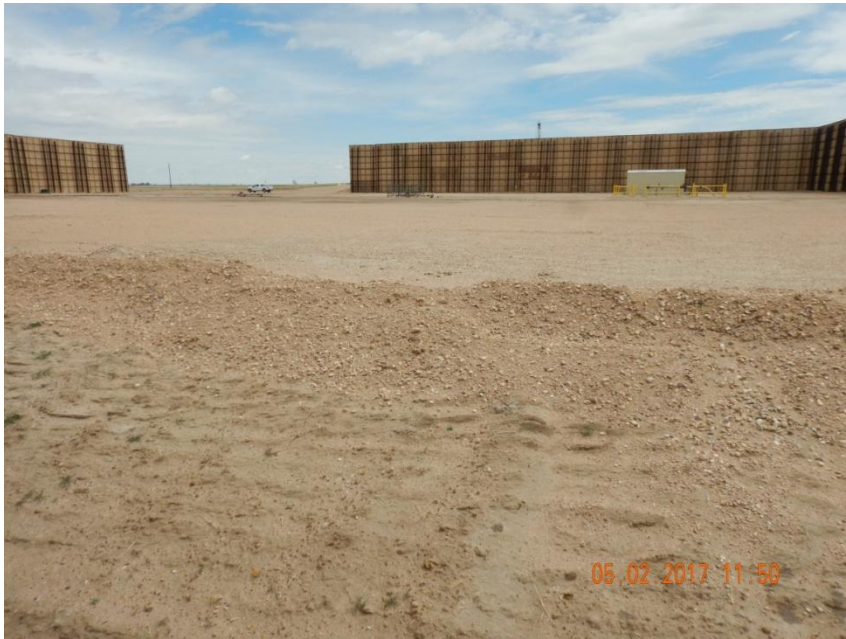
Photo 5. Photo taken from the western location, facing East. Gravel berm has been constructed around the outer well pad area and fill slopes have been properly tracked.
