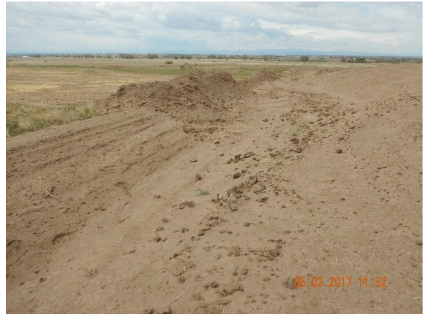
Photo 6. Photo taken from the south perimeter of the location, facing West. Appears soil material has been moved and because of flow line activity. Unconsolidated soil material needs to be stabilized to prevent sediment discharge off location.
