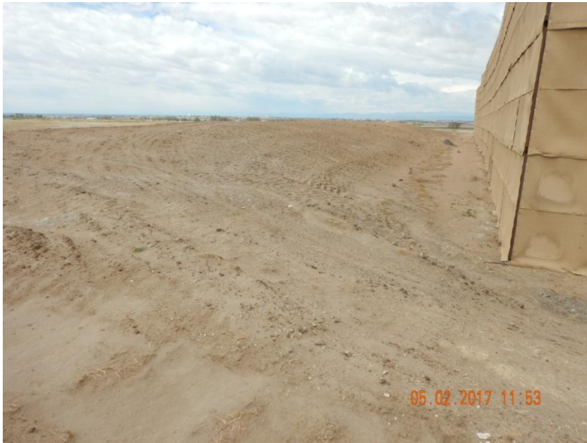
Photo 7. Photo taken from the southeastern location, facing West. Topsoil has been salvaged, stored and temporarily stabilized along the southern perimeter of the location.
