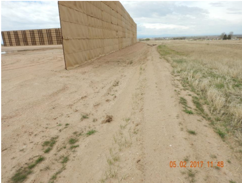
Photo 1. Photo taken from the northeast perimeter of the location, facing West. Ditch and berm BMP has been installed around the entire perimeter of the location in conjunction with other BMPs and appears to be properly functioning.
