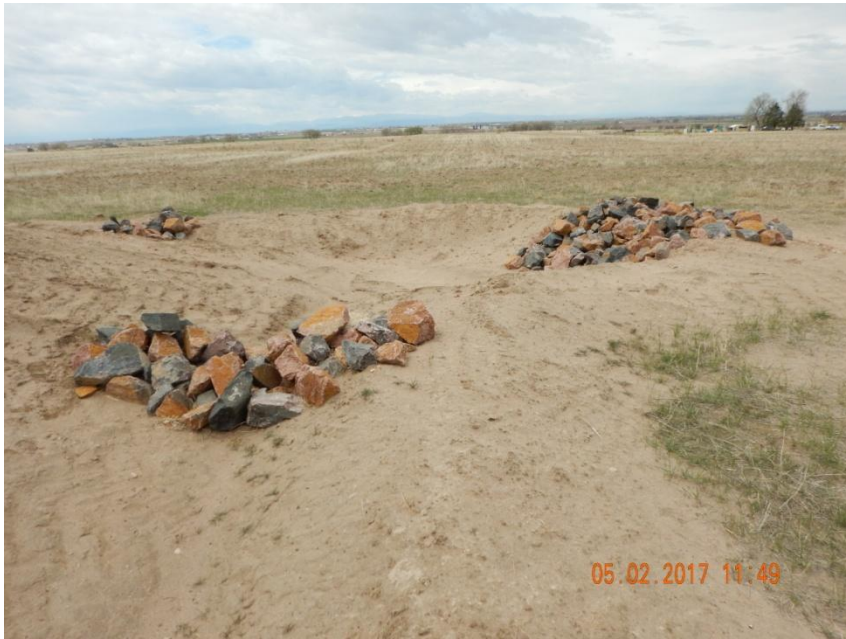
Photo 3. Photo taken from the northwest perimeter of the location, facing West. Sediment trap has been installed with both inlet and outlet protection.
