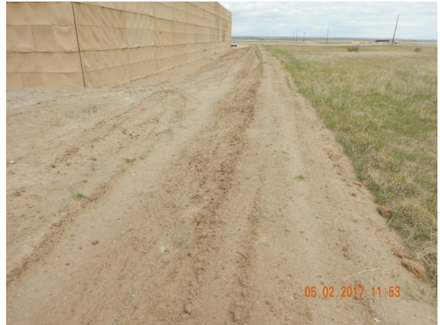
Photo 8. Photo taken from the southeast perimeter of the location, facing North. Ditch and berm BMP has been installed.
