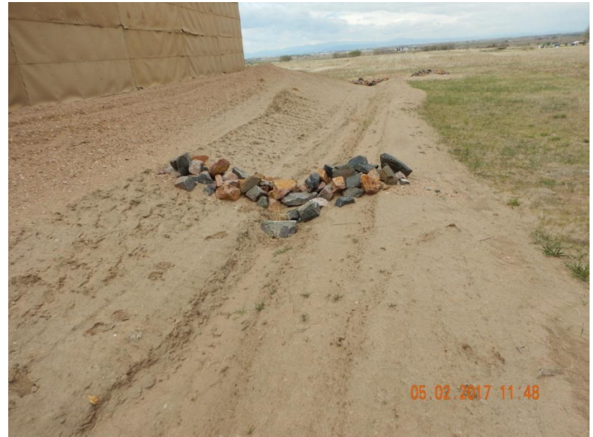
Photo 2. Photo taken from the northwestern perimeter of the location, facing West. Ditch and berm BMP has been installed in conjunction with check dams prior to the sediment trap.
