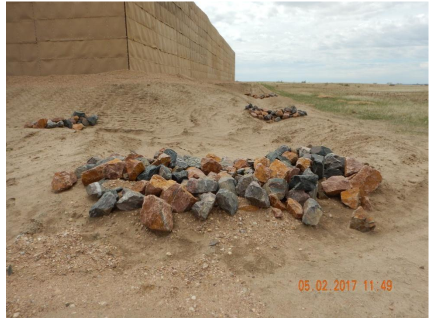
Photo 4. Photo taken from the northwest perimeter of the location, facing South. Sediment trap has been installed with both inlet and outlet protection, as well as check dams.
