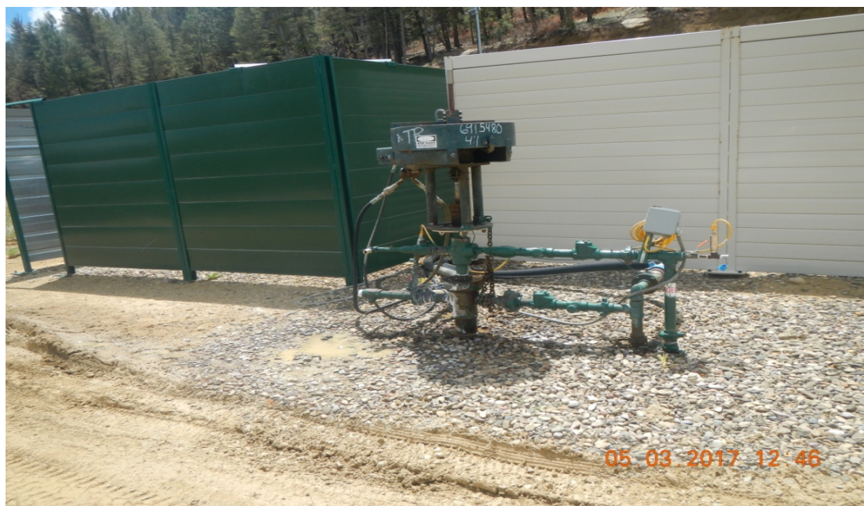
photo 3: There is a slow dripping water leak at the well head.
