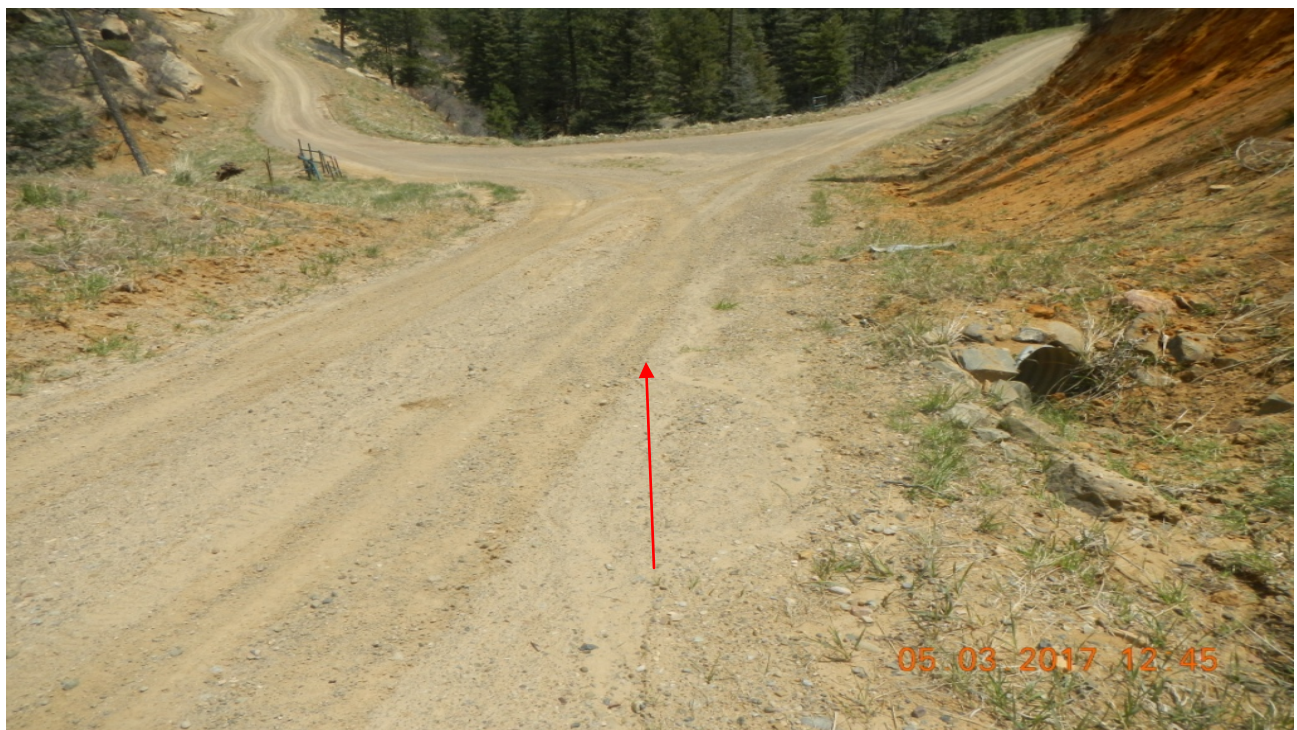
photo 2: Facing back toward the east at the access road. There are signs stormwater is draining down the road instead of toward the culvert. The water is pooling at the bottom of the road.
