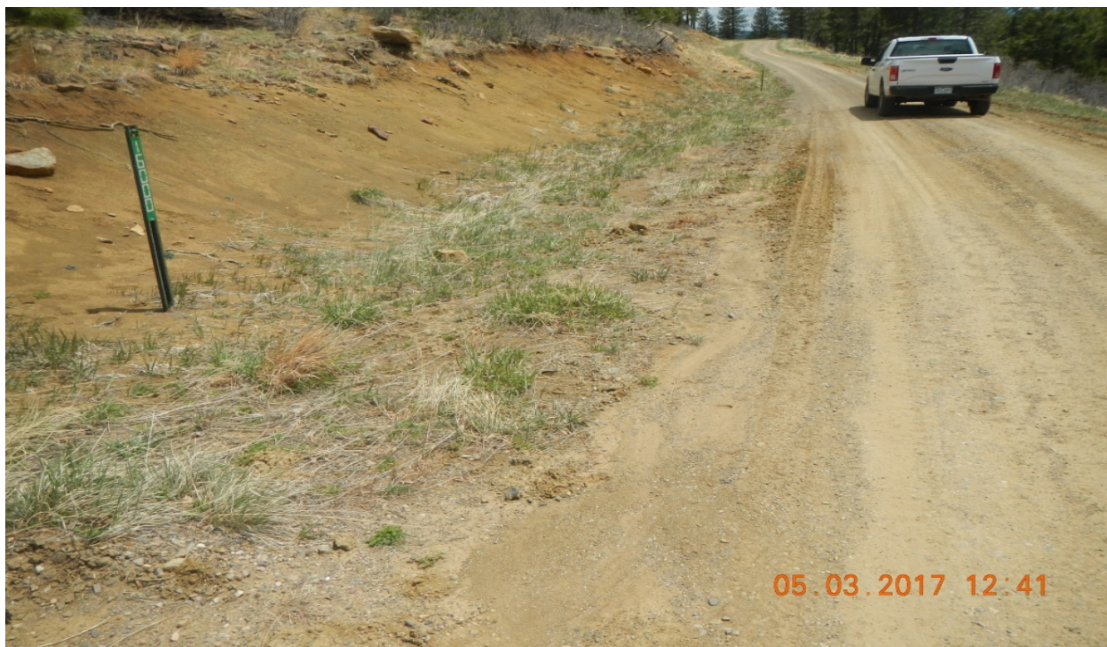
photo 5: Approximate Lat/Long:37.22408,-104.94292. Sediment has filled into the drainage ditch which is not allowing stormwater to flow toward the culvert.
