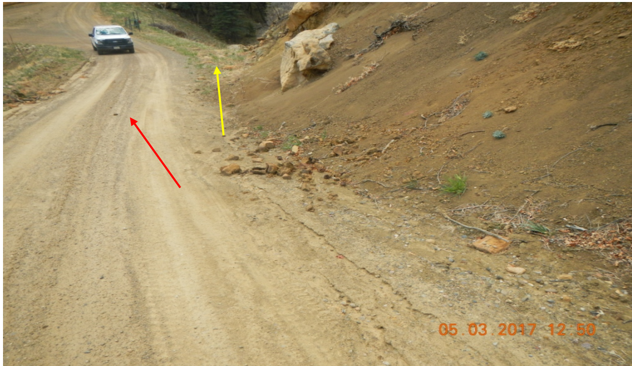
photo 3: Approximate Lat/Long:37.22630,-104.94464. Stormwater is flowing and pooling on the road in the direction of the red arrow. The diversion ditch along the side of the road is filled in and not draining as it should in the direction shown by the yellow arrow.
