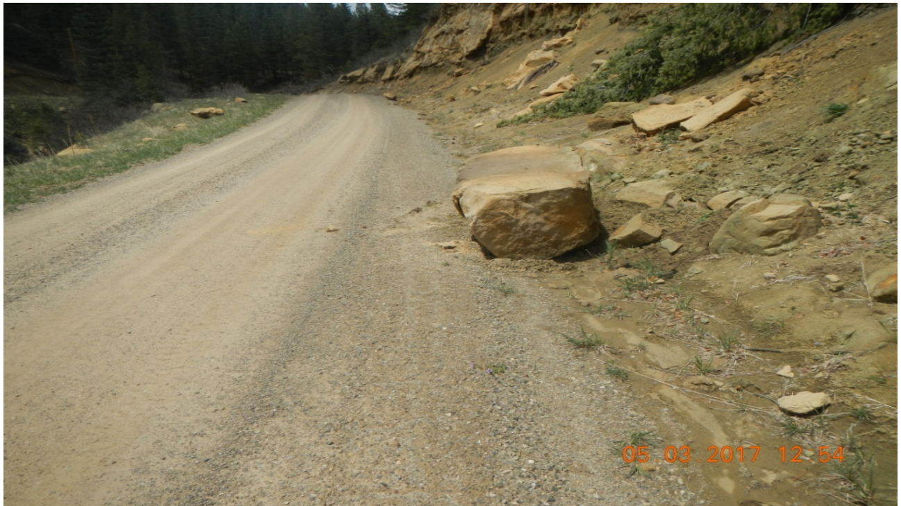
photo 1: Facing west along main road at approximate Lat/Long: 37.22886,-104.94239. A boulder has fallen near the side of the road which will restrict stormwater flow.
