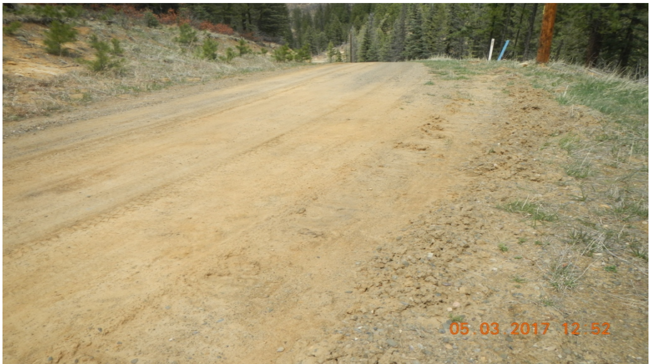
photo 2: The gravel has been scrapped of the road and there is little gravel that remains at this area along the main road at approximate Lat/Long:37.22886,-104.94272.
