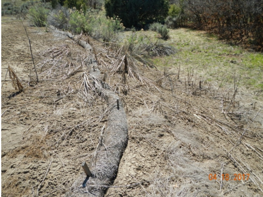
Photo 3: View of wattles in the western portion of the project area. These are filling with sediment and will soon need maintenance.
