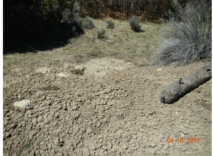
Photo 4: View of the edge of placed wattles exposed soils and evidence of sediment deposition below. Musk thistles are also growing in this portion of the project area.
