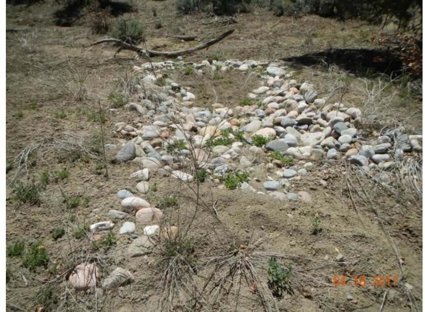
Photo 6: View of cobble rundown in the southwestern portion of the project area that is filling with sediment and needs maintenance.
