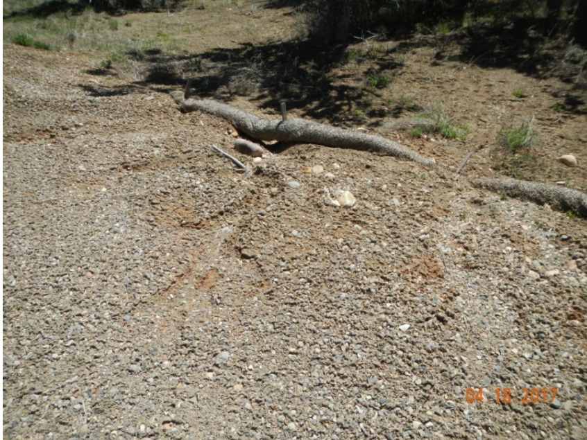
Photo 5: View of wattles in the southern portion of the project area that are not functioning and need repair or replacement.
