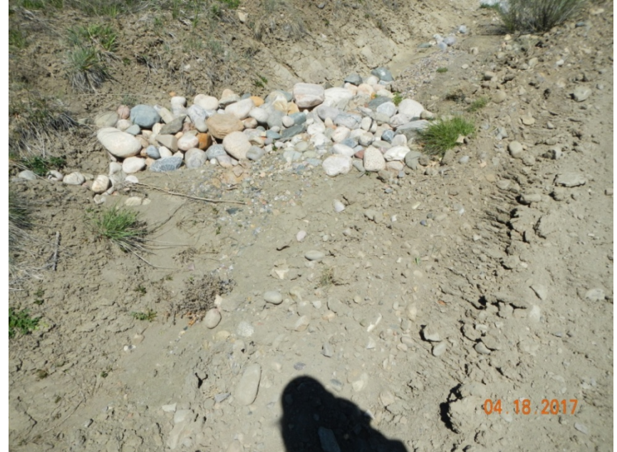
Photo 4: View of check dam that is largely full of sediment and needs maintenance.
