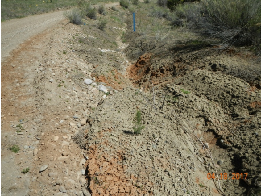
Photo 3: View of exposed soil and erosional channels forming along the southern edge of the access road at the well pad entrance.
