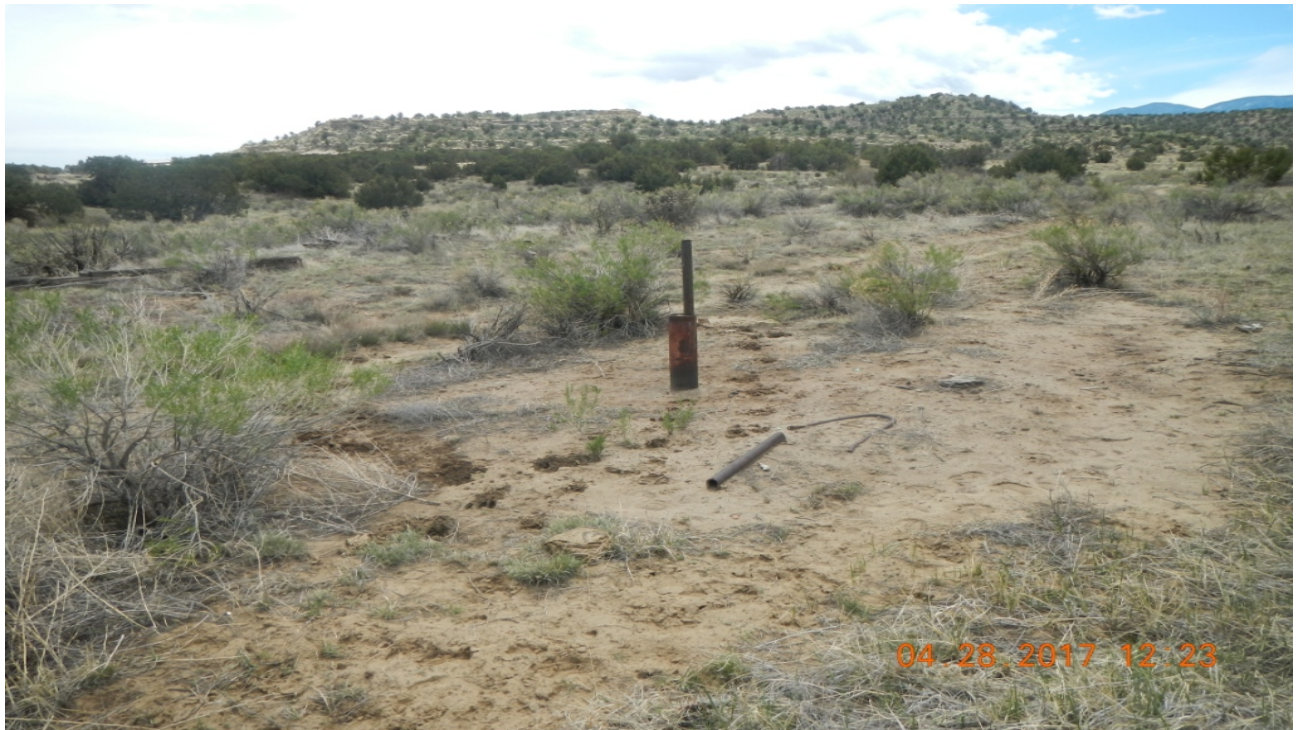
photo 1: Well casing at the location.
