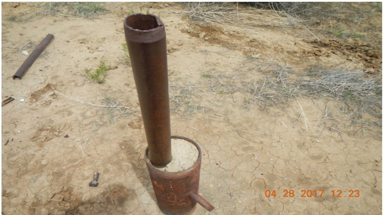
photo 2: View of casing which looks to be cemented.
