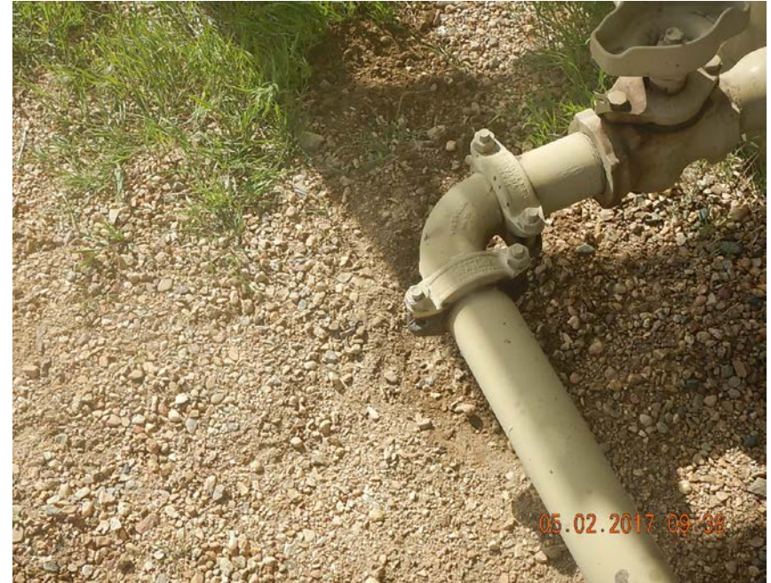
Photo 5: Stained soil removed
