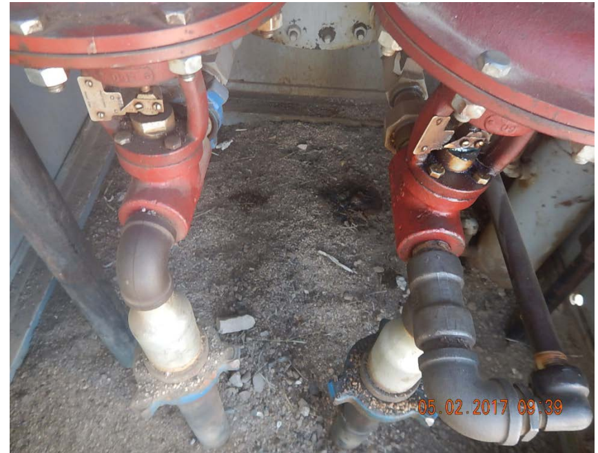
Photo 6: Stained soil removed, new stained soil in separator house
