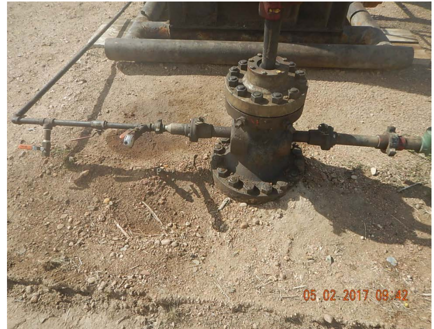
Photo 2: Stained soil at wellhead removed, stained soil near wellhead.
