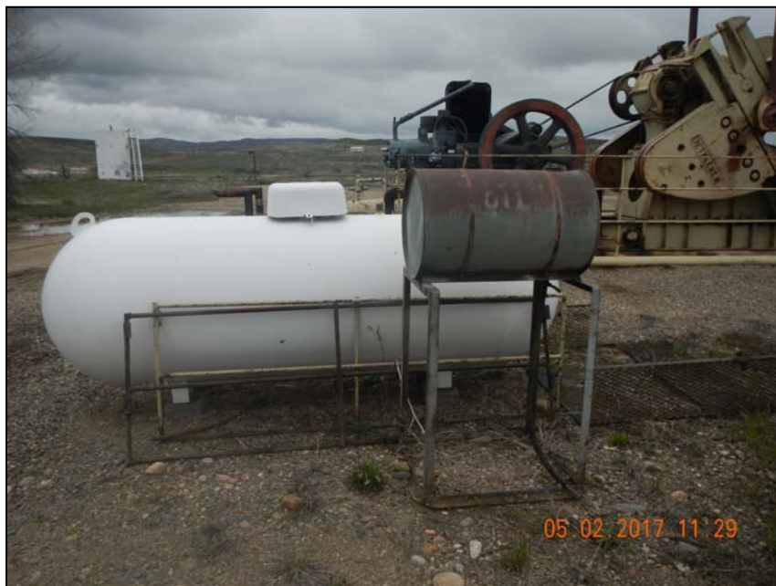
Photo 3. Unlabeled container with no secondary containment.
