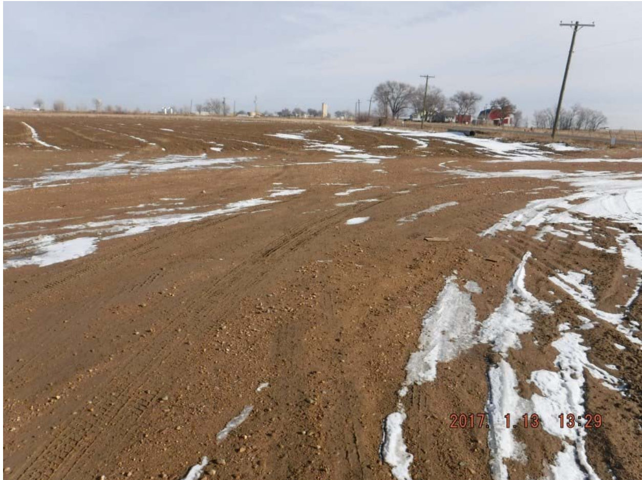
Photo of armored work area
