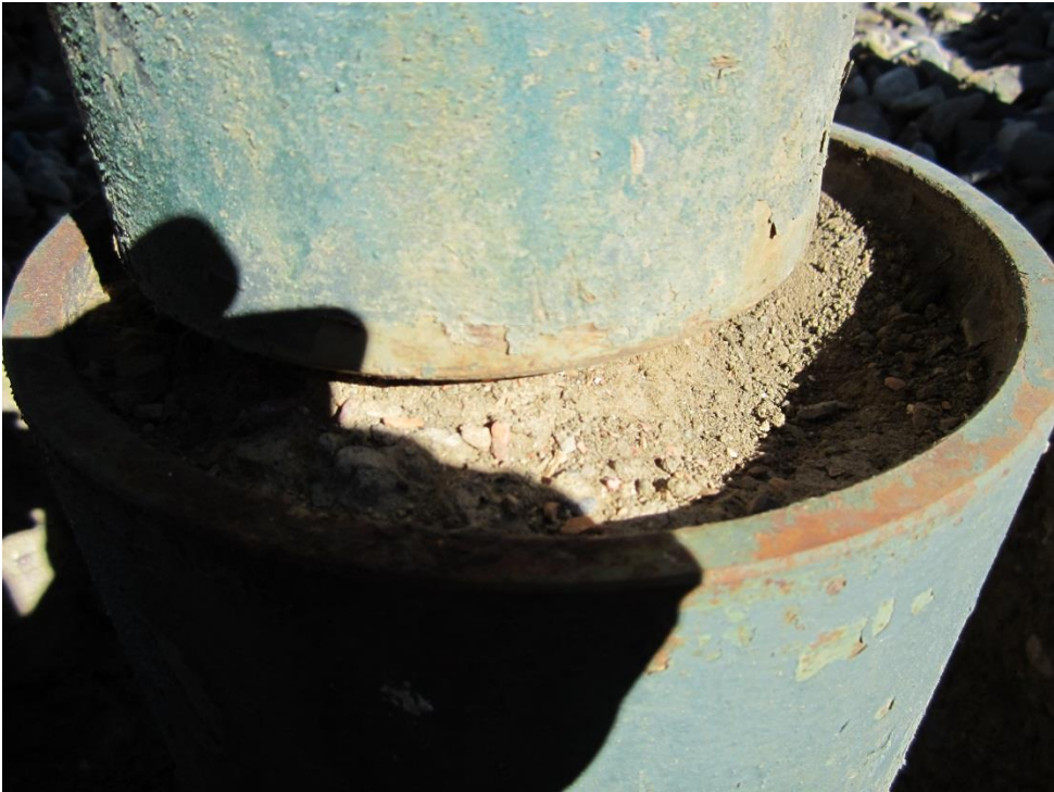
Surface Casing Photo – Dug out
