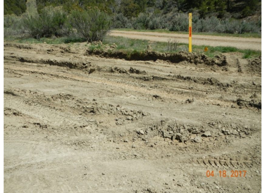
Photo 4: View of deep rutting and damaged vegetation from truck tires at the well pad entrance. This area needs stabilization.
