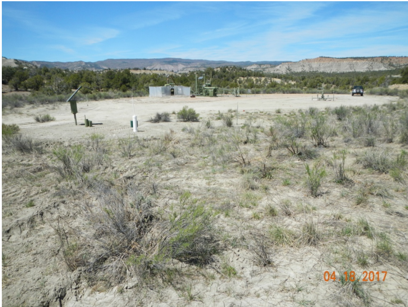
Photo 1: View of the project area from the southeastern corner facing center. Equipment has left deep ruts and damaged vegetation within the southeastern portion of the project area (lower left corner of photo).
