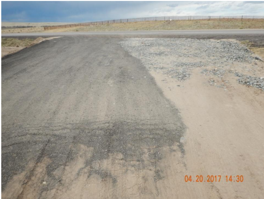
Photo 1. Photo taken from the entrance of the location just off Quincy Ave., facing North. Tracking pad material installed but does not appear to be consistently installed throughout the entrance. However, crushed asphalt has been installed along the entire access road which should minimize sediment discharge via vehicle tracking.
