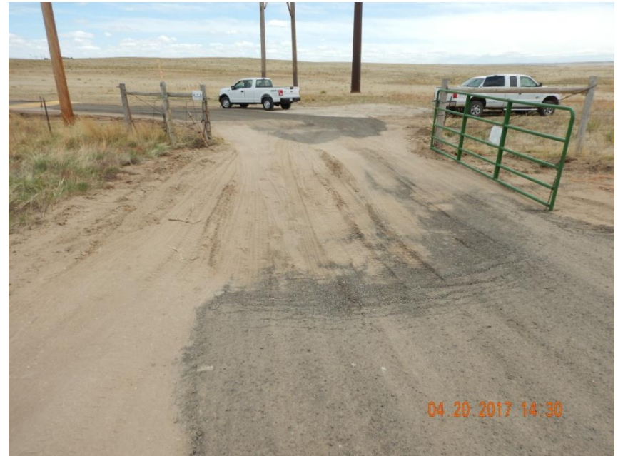
Photo 2. Photo taken from the entrance of the location just off Quincy Ave., facing South. Tracking pad material installed but does not appear to be consistently installed throughout the entrance. However, crushed asphalt has been installed along the entire access road which should minimize sediment discharge via vehicle tracking.
