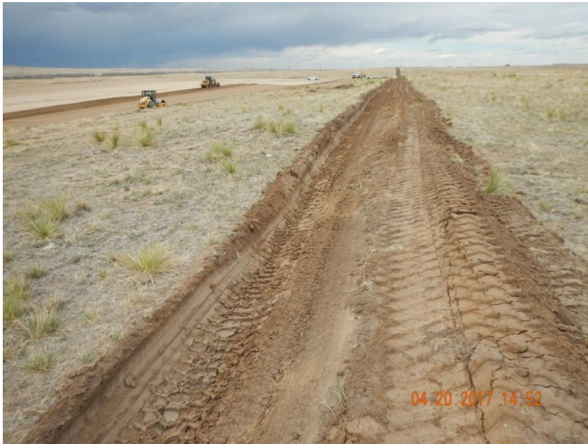
Photo 15. Photo taken from the southeast perimeter of the well pad location, facing North. A ditch and berm BMP has been installed along the entire perimeter of the location.
