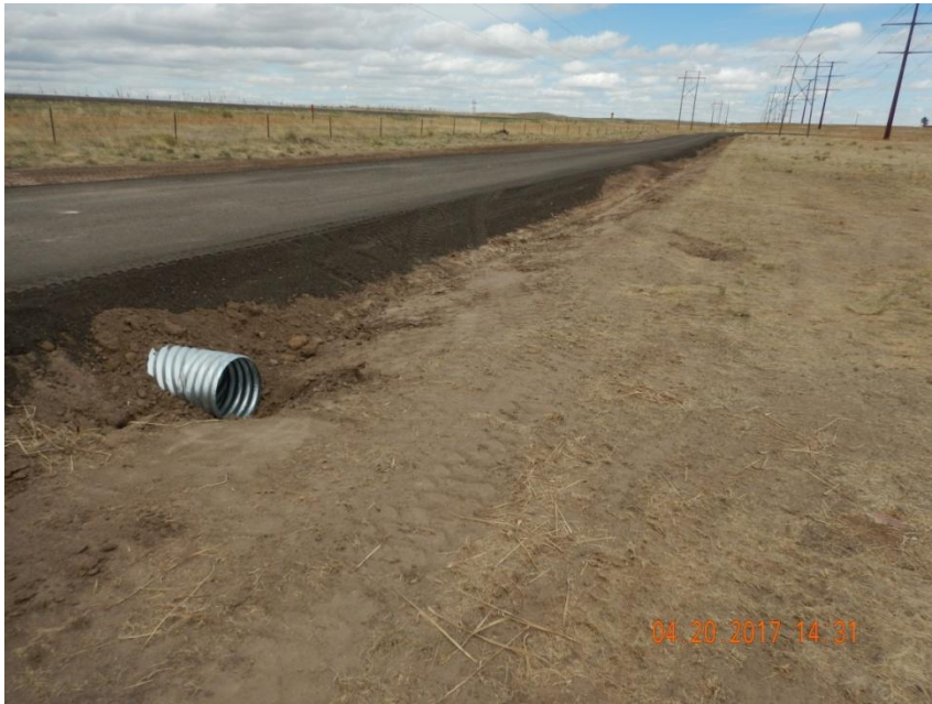
Photo 5. Photo taken from the cattle guard and culvert, facing East. Photo illustrates the crushed asphalt that has been installed along the access road.
