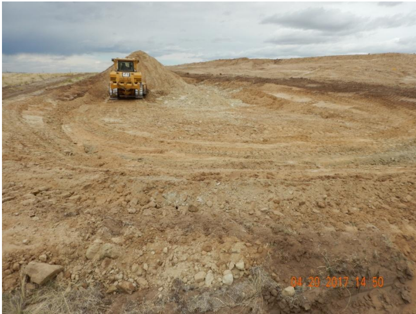
Photo 13. Photo taken from the southwest perimeter of the well pad location, facing North. Operator in the process of installing a retention area for stormwater control. At the time of this inspection, it was unclear how stormwater runoff will be directed to the retention area from the ditch and berm BMP.
