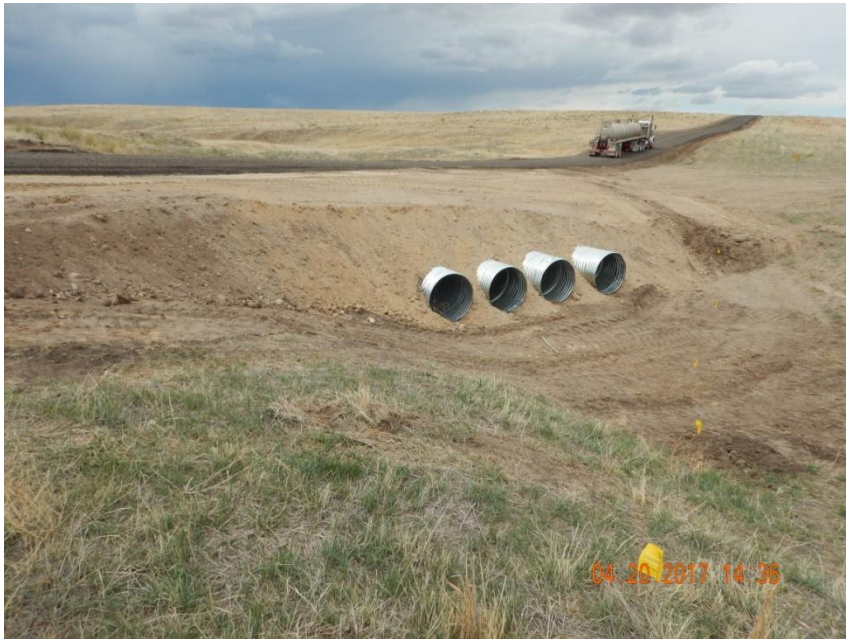
Photo 7. Photo taken along a drainage area on the east side, facing Northwest. Culverts have been installed along the drainage area. This area has potential for erosion along the fill slopes and stormwater runoff from the access road. Did not observe any erosion control BMPs along this area at the time of this inspection.
