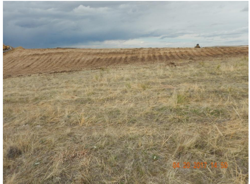
Photo 14. Photo taken from the southern location, facing North. Fill slope appears to be properly tracked.
