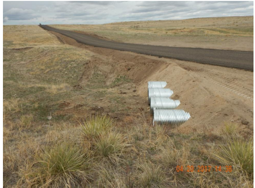
Photo 8. Photo taken along a drainage area on the west side, facing Northeast. Culverts have been installed along the drainage area. This area has potential for erosion along the fill slopes and stormwater runoff from the access road. Did not observe any erosion control BMPs along this area at the time of this inspection.
