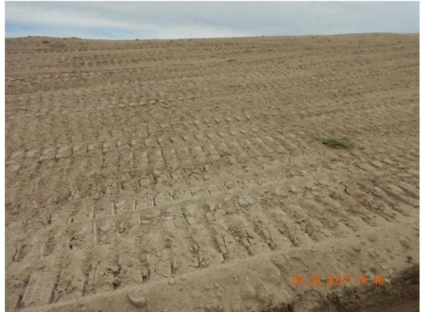
Photo 10. Photo taken along the northern fill slope, facing South. Fill slope has not been tracked perpendicular to the slope which could increase potential erosion along this area.
