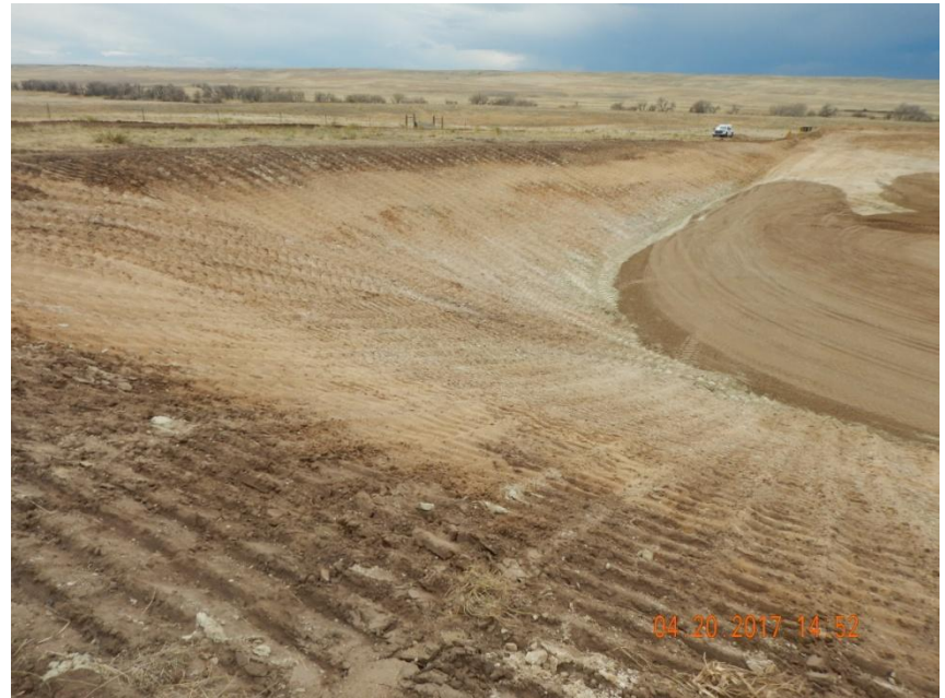
Photo 16. Photo taken from the southeast cut slope of the well pad location, facing West. Cut slope along the entire well pad area appears to be properly tracked.
