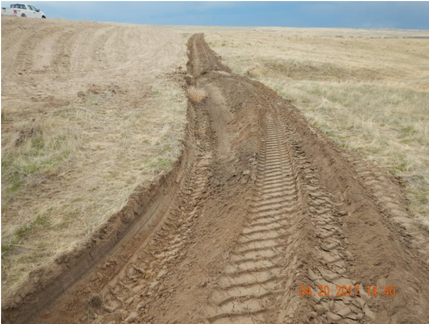
Photo 9. Photo taken from the northeast perimeter of the well pad location, facing West. A ditch and berm BMP has been installed along the entire perimeter of the location.
