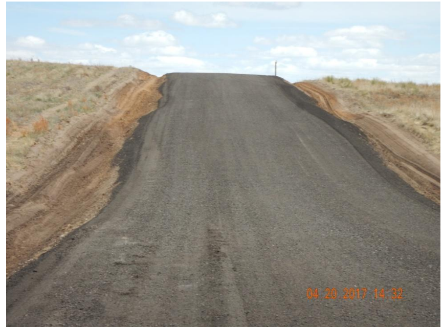
Photo 6. Photo taken from along the access road, facing South. Photo illustrates the crushed asphalt that has been installed along the access road. Also, it appears a diversion ditch has been installed along both sides of the entire access road.
