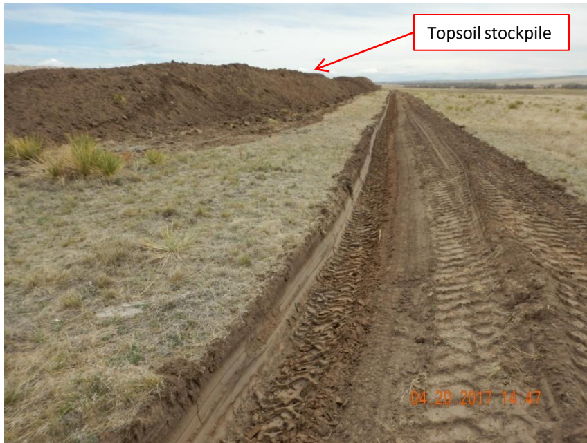
Photo 11. Photo taken from the northwest perimeter of the well pad location, facing South. A ditch and berm BMP has been installed along the entire perimeter of the location.
