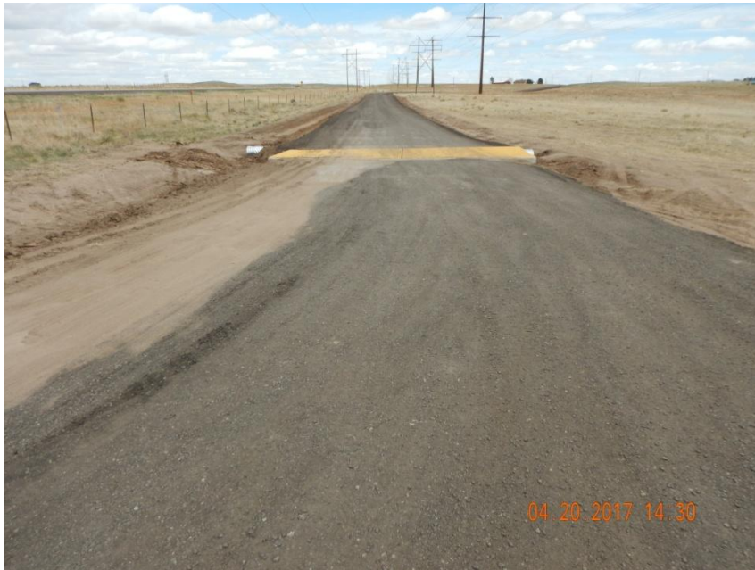
Photo 3. Photo taken just beyond the entrance off Quincy Ave., facing East. Cattle guard installed in conjunction with a culvert. Crushed asphalt has been installed along the entire access road which should minimize sediment discharge via vehicle tracking.
