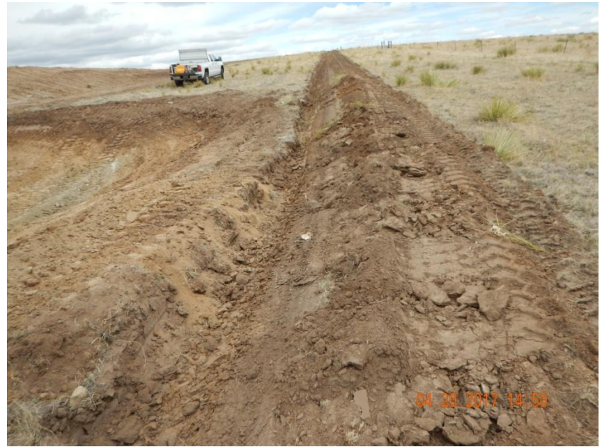
Photo 12. Photo taken from the southwest perimeter of the well pad location, facing East. A ditch and berm BMP has been installed along the entire perimeter of the location.
