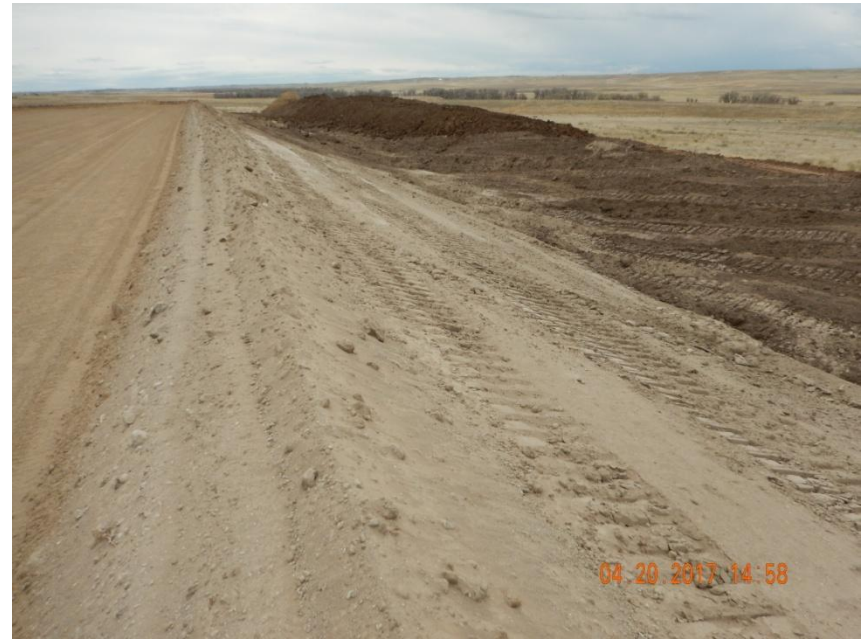
Photo 18. Photo taken from the western fill slope of the well pad location, facing North. Fill slope has not been tracked perpendicular to the slope which could increase potential erosion along this area.
