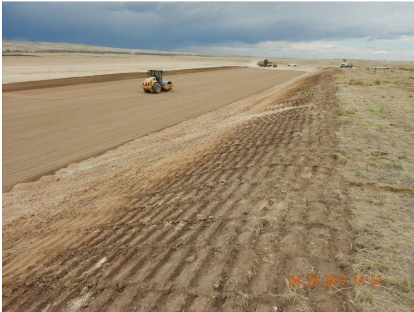
Photo 17. Photo taken from the southeast cut slope of the well pad location, facing North. Cut slope along the entire well pad area appears to be properly tracked.
