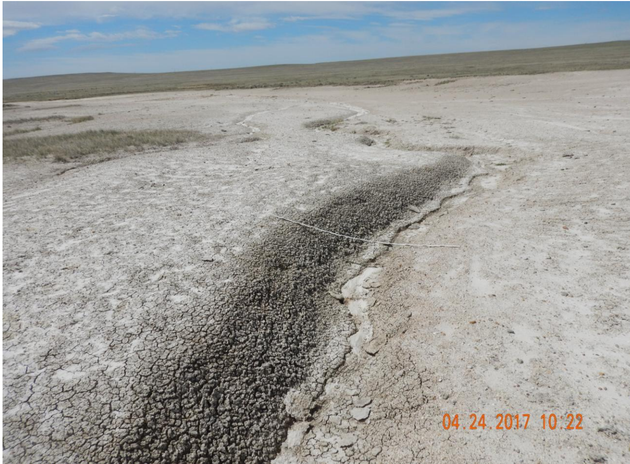
Photo 10: Photo taken from within the salt kill. Photo shows large gully that has formed due to improper site stabilization. 6 foot measuring stick for reference.
