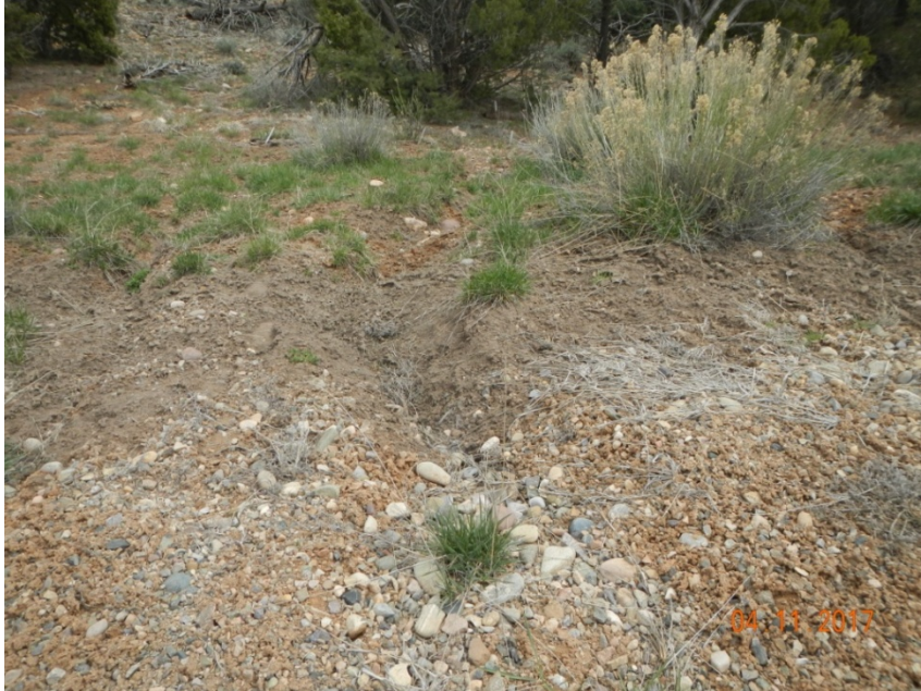
Photo 5: View of erosional channel approximately 2 feet wide and 1.5 feet deep within the eastern portion of the project area.
