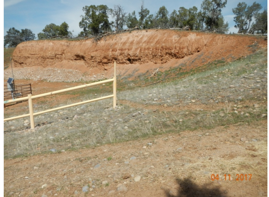
Photo 2: View of the eastern portion of the project area from the southeastern corner facing northward. Revegetation is largely comprised of grasses such as dropseed ( Sporobolus sp.). Much of the revegetation is comprised of annual weeds such as cheatgrass ( Bromus tectorum ) and stork's bill ( Erodium cicutarium ). Northeastern cut-slope is too steep to support vegetation.
