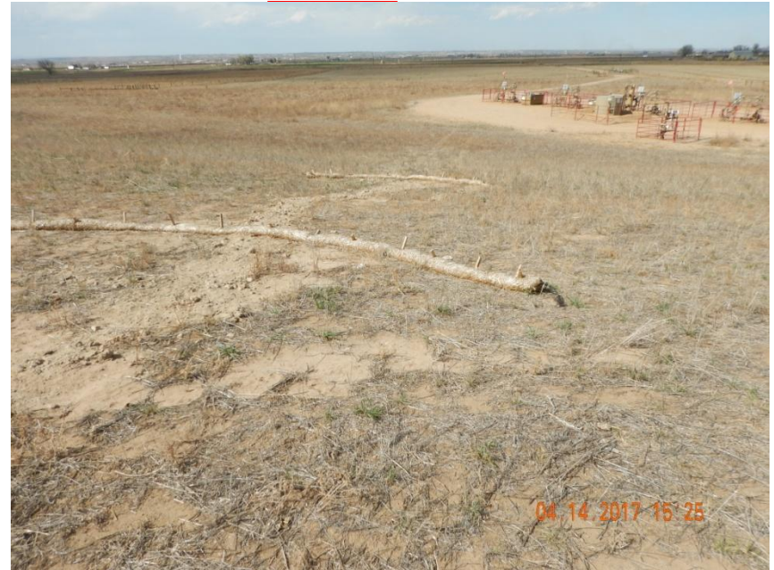
Photo 16. Photo taken from the previous photo location, facing North. A series of wattle BMPs have been installed to control run-on onto the interim area. Portions where erosion was previously observed still lack germination growth.
