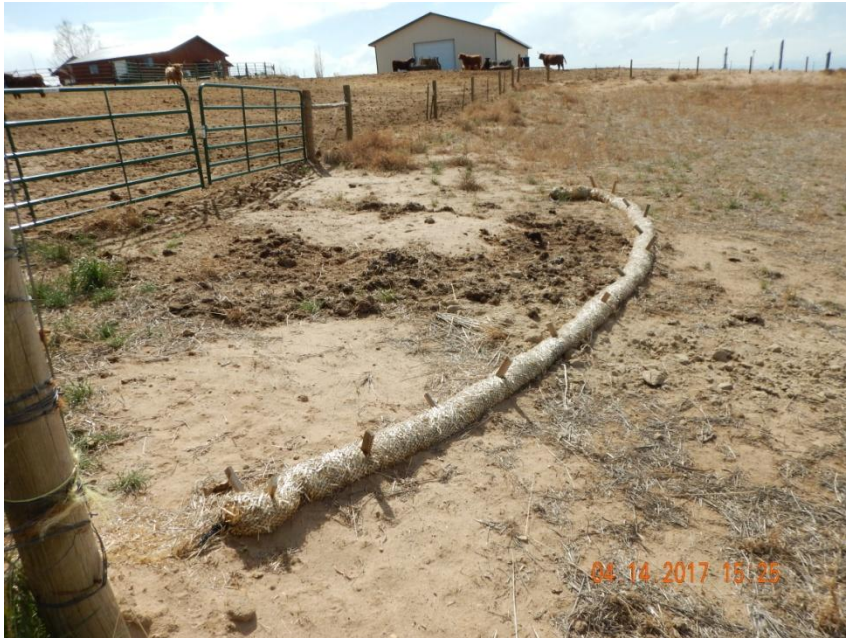
Photo 15. Photo taken from the southern location, facing West. Wattle BMPs installed to control run-on onto the interim area. Portions where erosion was previously observed still lack germination growth.
