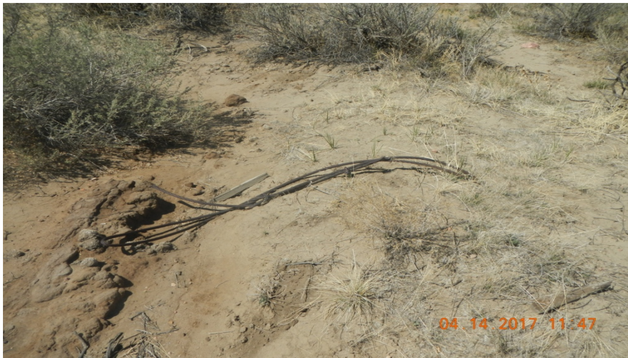
photo 3: Guyline anchor remains at the northwest corner of the location.
