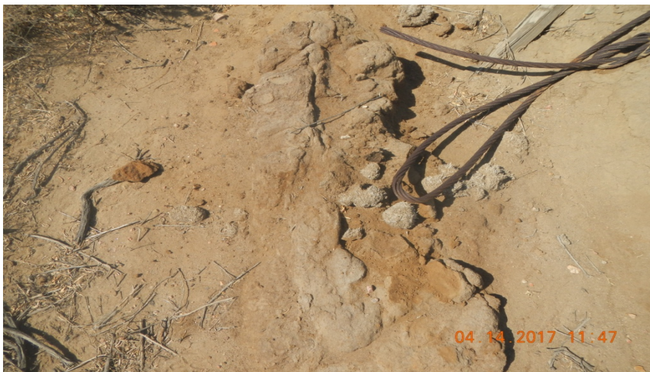
photo 4: The soil around the northwest guyline anchor appears to have oil stained soils.
