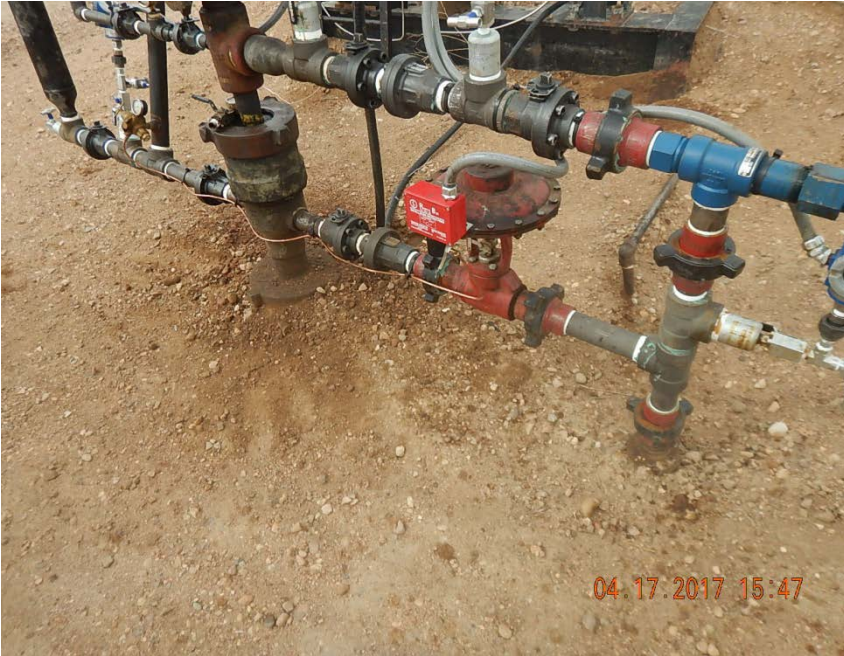
Photo 3: Stained soil at wellhead
