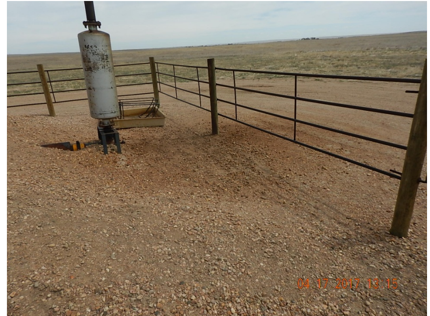
Photo 4: Stained soil at Ajax exhaust
