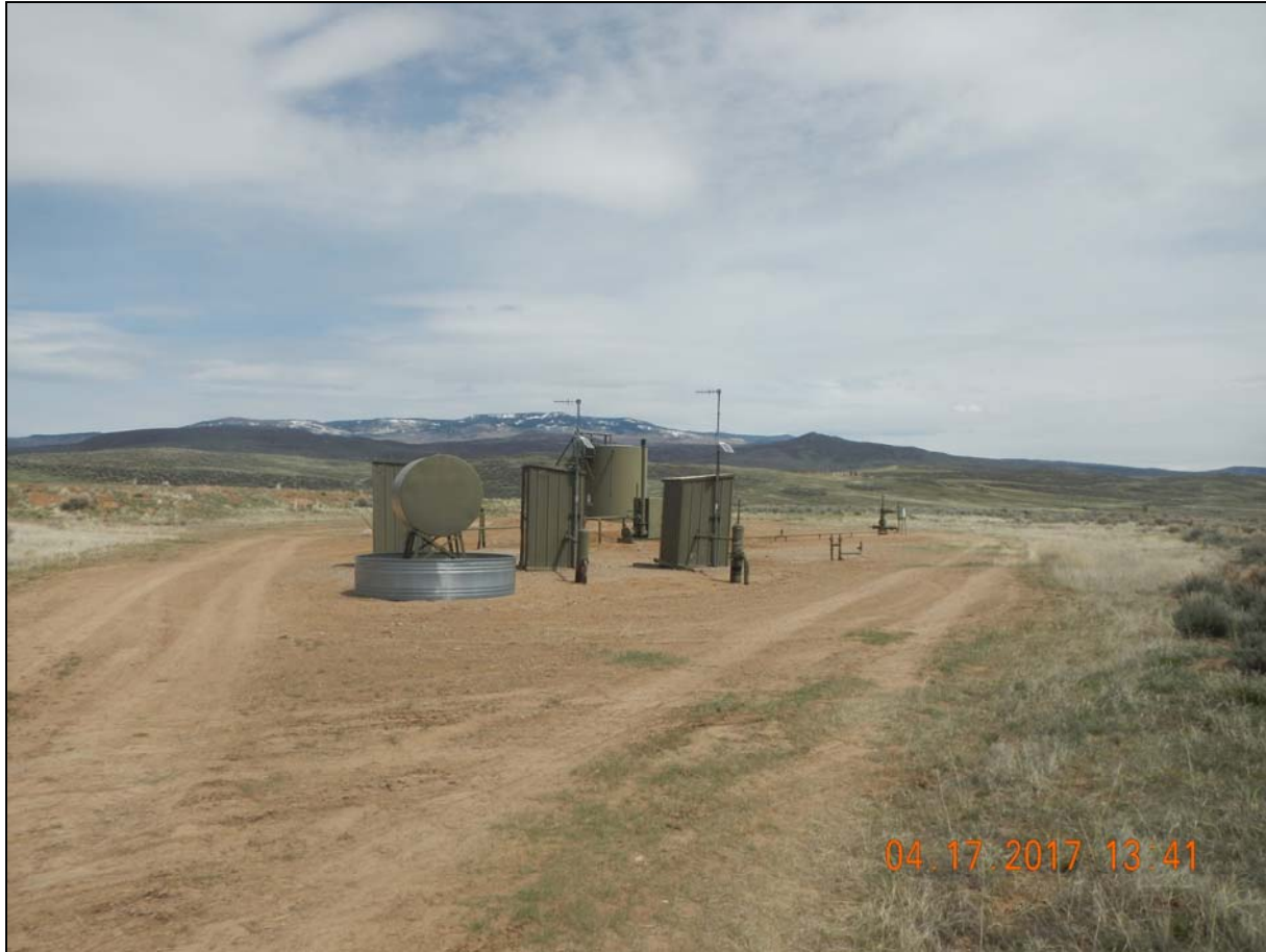
Photo 1. View at entrance to location facing east.
