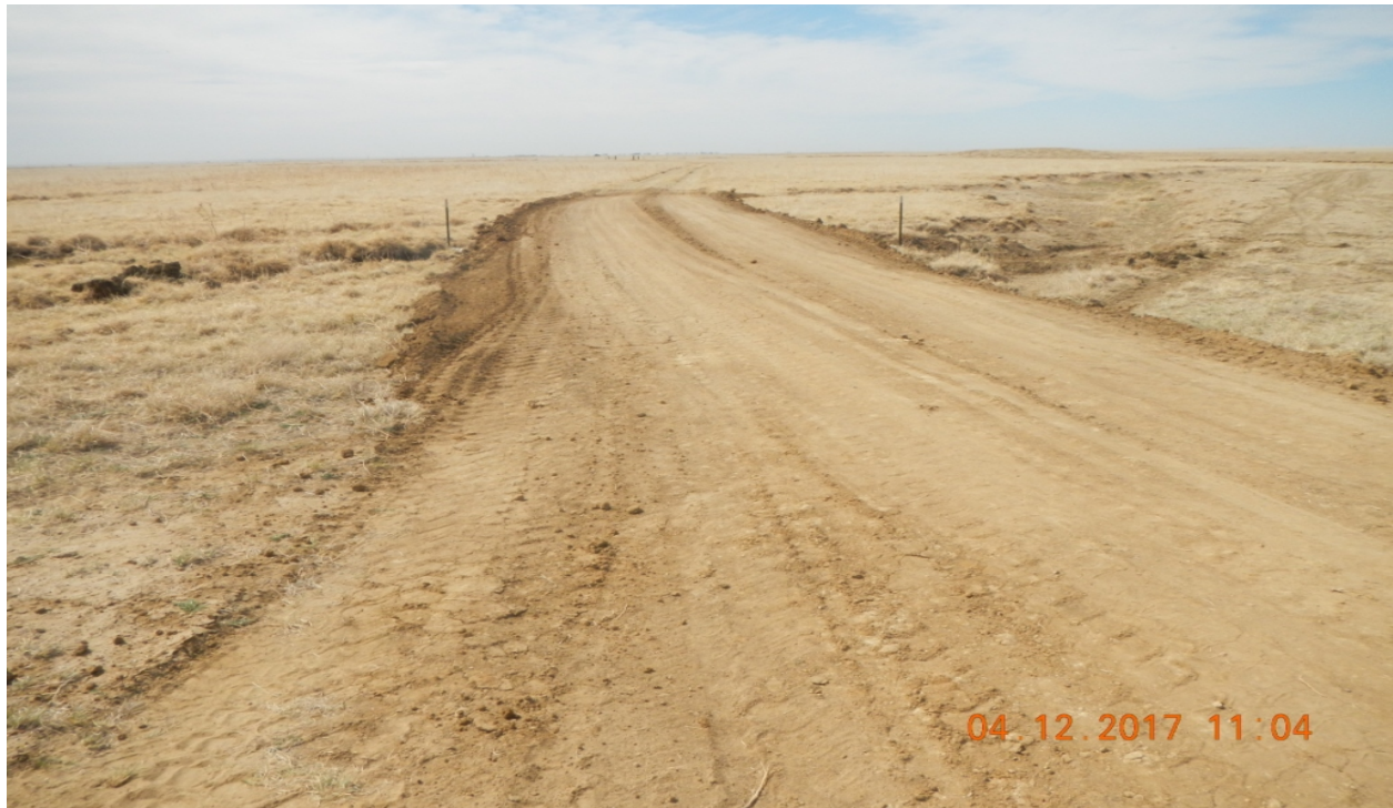
photo 5: Facing south, culverts are installed and material from the borrow area is placed over the culverts.
