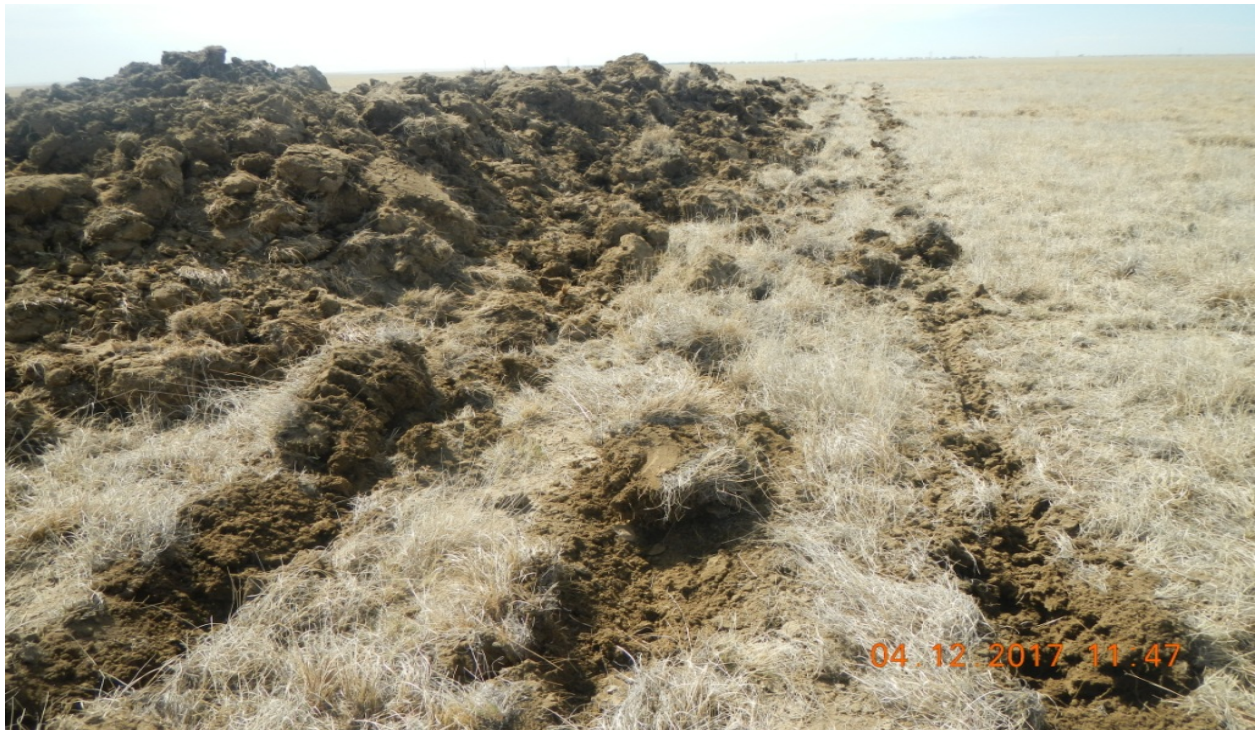
photo 9: Facing south toward topsoil pile. Surface roughening has occurred around the perimeter.
