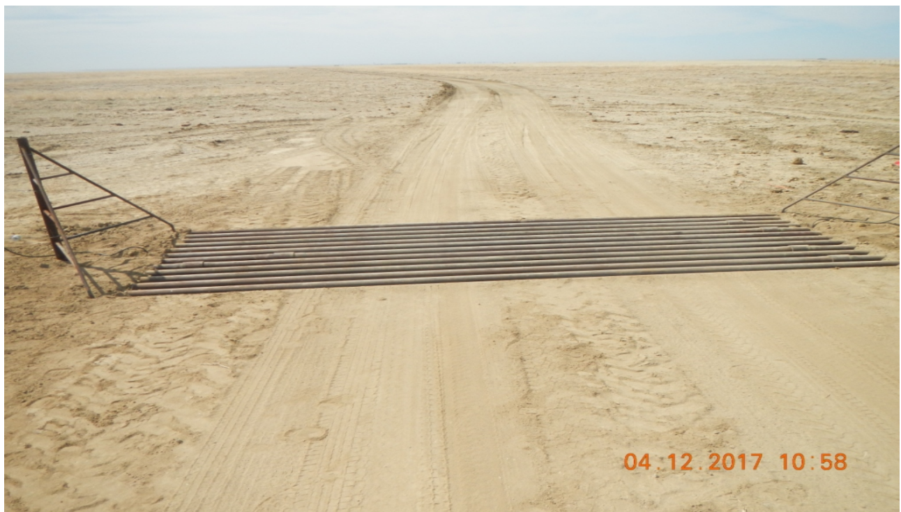
photo 2: Further south along the road, a second cattle guard is installed.
