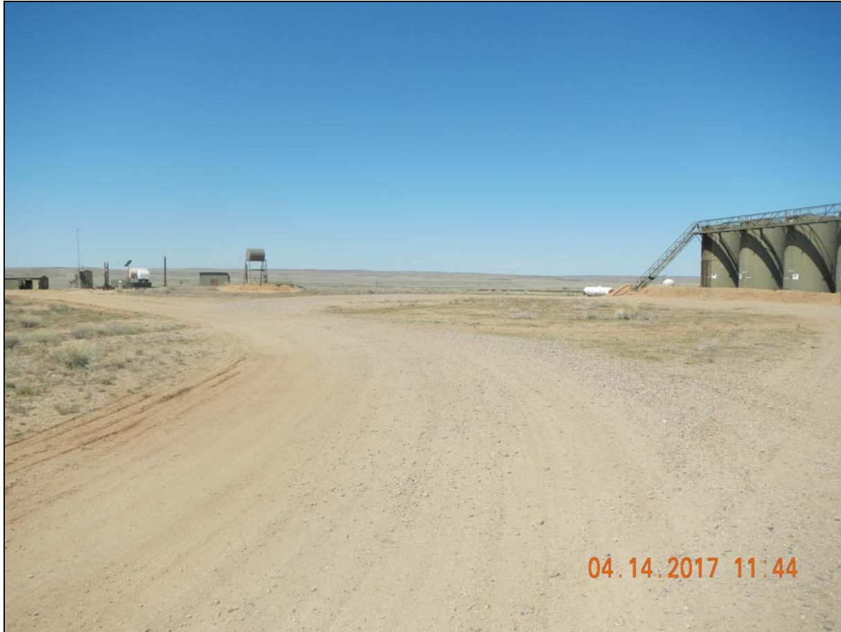
Photo 1. View at entrance to location facing southwest.
