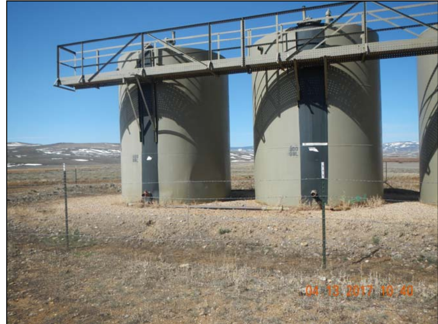
Photo 2. Missing tank labels.
