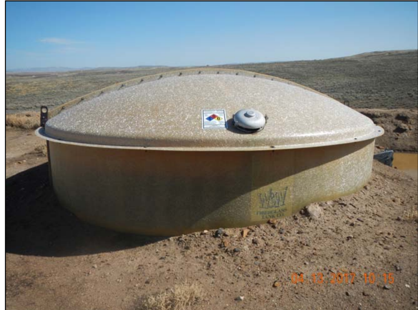
Photo 4. No capacity on produced water tank.
