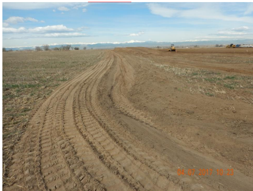
Photo 4. Photo taken from the southeast location, facing West. Ditch and berm BMP installed around the perimeter of location. Also, location is dominated by sandy soils so a tackifier is recommended to stabilize all disturbed areas to control for wind erosion.
