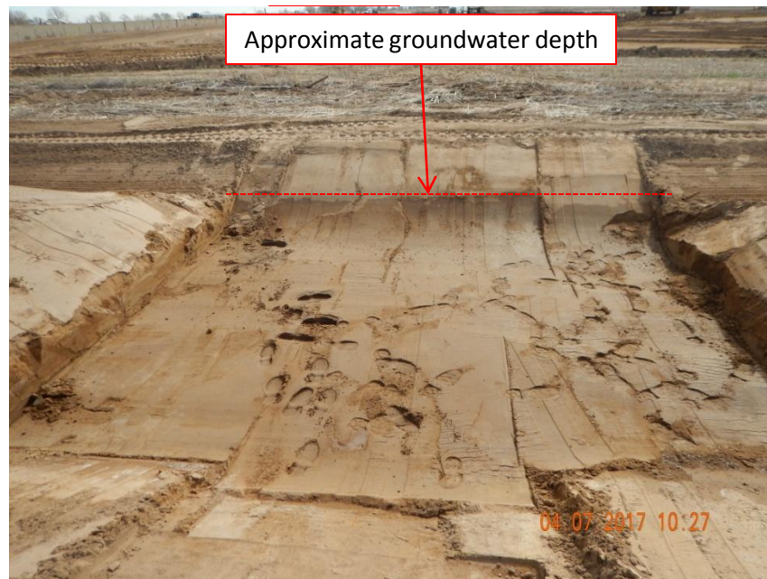
Photo 8. Photo taken from inside the western sediment trap. Shallow groundwater has been encountered while constructing the sediment trap. Approximate groundwater depth is illustrated with the line. Operator needs to construct BMPs in such a manner that would not have direct impact to groundwater.
