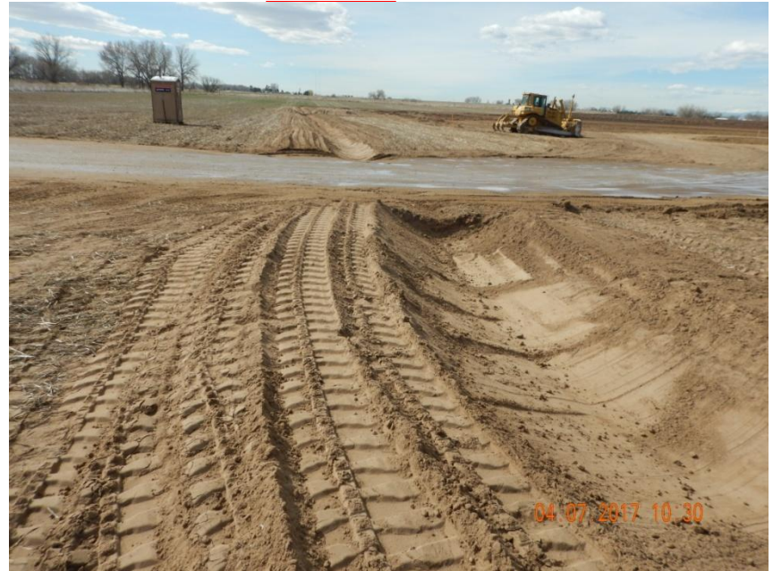
Photo 10. Photo taken from the northeast location, facing South. Ditch and berm BMP installed around the perimeter of location. Also, location is dominated by sandy soils so a tackifier is recommended to stabilize all disturbed areas to control for wind erosion.
