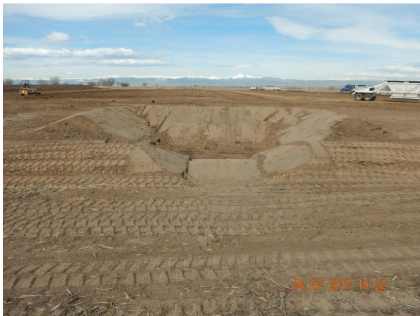
Photo 3. Photo taken from the eastern location, facing West. Sediment trap installed and IN-PROCESS of being completed (i.e., outlet still needs to be stabilized). Also, location is dominated by sandy soils so a tackifier is recommended to stabilize all disturbed areas to control for wind erosion.
