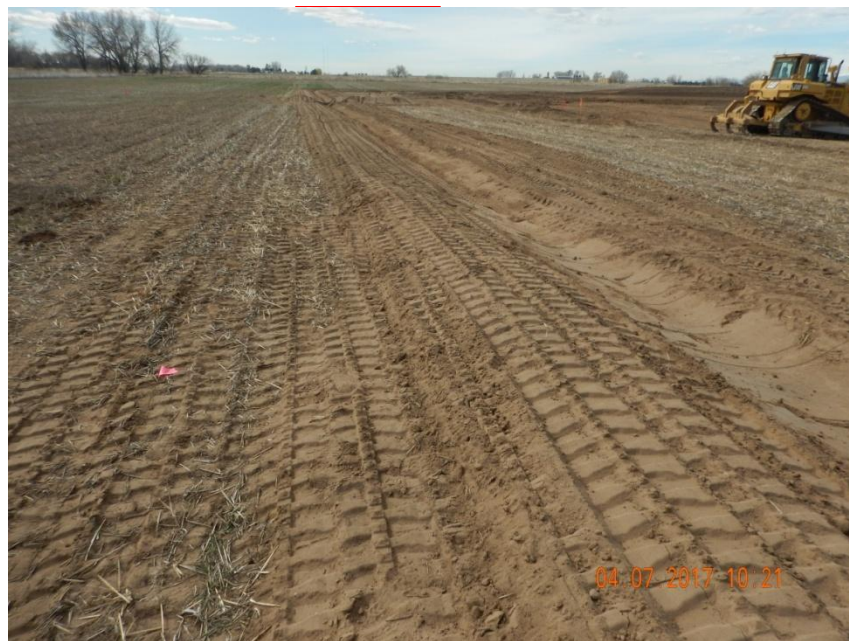
Photo 2. Photo taken from the northeast location, facing South. Ditch and berm BMP installed around the perimeter of location. Also, location is dominated by sandy soils so a tackifier is recommended to stabilize all disturbed areas to control for wind erosion.
