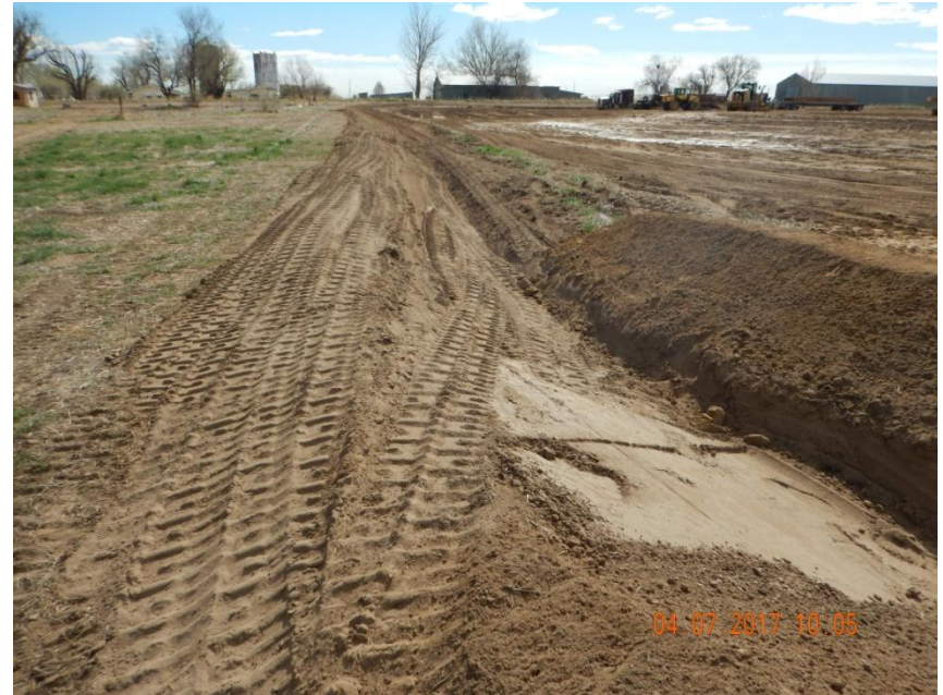
Photo 8. Photo taken from the northwest location, facing East. Ditch and berm BMP installed around the perimeter of location. Also, location is dominated by sandy soils so a tackifier is recommended to stabilize all disturbed areas to control for wind erosion.
