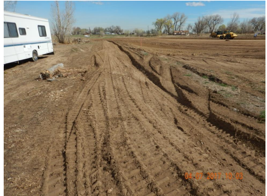
Photo 4. Photo taken from the southwest location, facing North. Ditch and berm BMP installed around the perimeter of location. Also, location is dominated by sandy soils so a tackifier is recommended to stabilize all disturbed areas to control for wind erosion.
