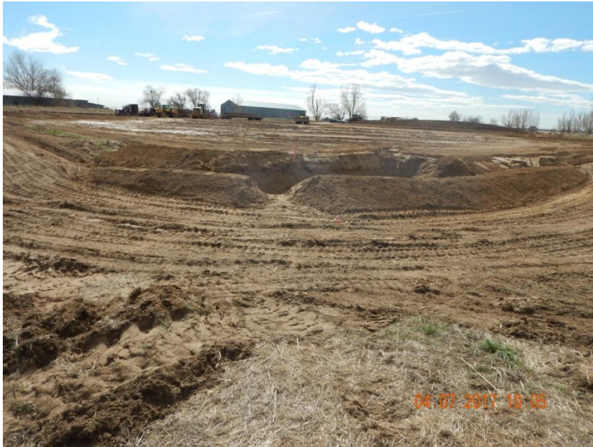
Photo 7. Photo taken sediment trap, facing Southeast. Sediment trap installed and IN-PROCESS of being completed (i.e., outlet still needs to be stabilized).
