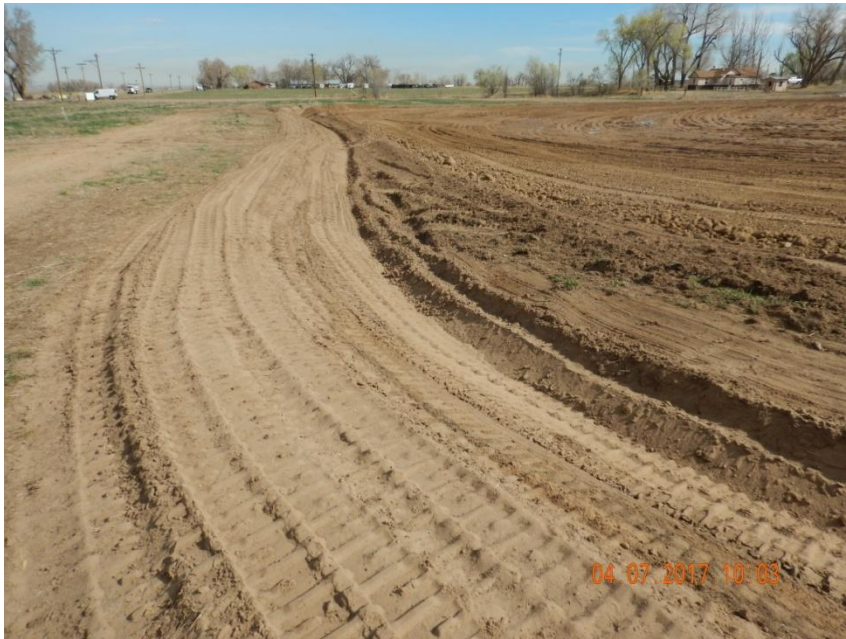
Photo 5. Photo taken from the western location, facing North. Ditch and berm BMP installed around the perimeter of location. Also, location is dominated by sandy soils so a tackifier is recommended to stabilize all disturbed areas to control for wind erosion.
