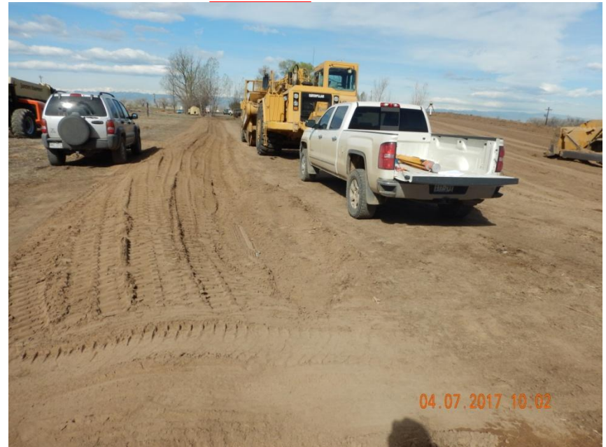
Photo 2. Photo taken from the southeastern location, facing West. Ditch and berm BMP installed around the perimeter of location. Also, location is dominated by sandy soils so a tackifier is recommended to stabilize all disturbed areas to control for wind erosion.
