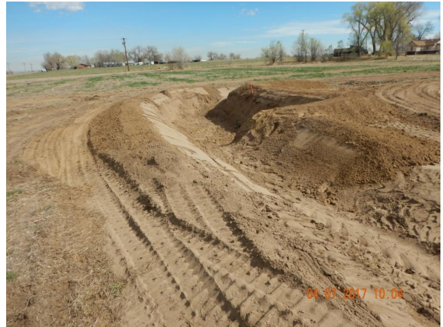
Photo 6. Photo taken from the northwest location, facing North. Sediment trap installed and IN-PROCESS of being completed (i.e., outlet still needs to be stabilized). Also, location is dominated by sandy soils so a tackifier is recommended to stabilize all disturbed areas to control for wind erosion.
