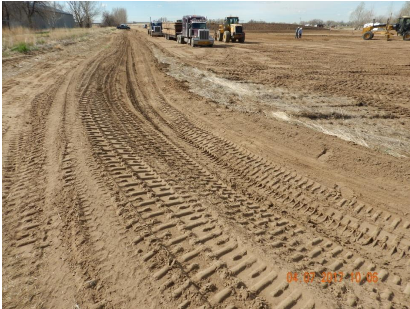
Photo 9. Photo taken from the northeast location, facing South. Ditch and berm BMP installed around the perimeter of location. Also, location is dominated by sandy soils so a tackifier is recommended to stabilize all disturbed areas to control for wind erosion.
