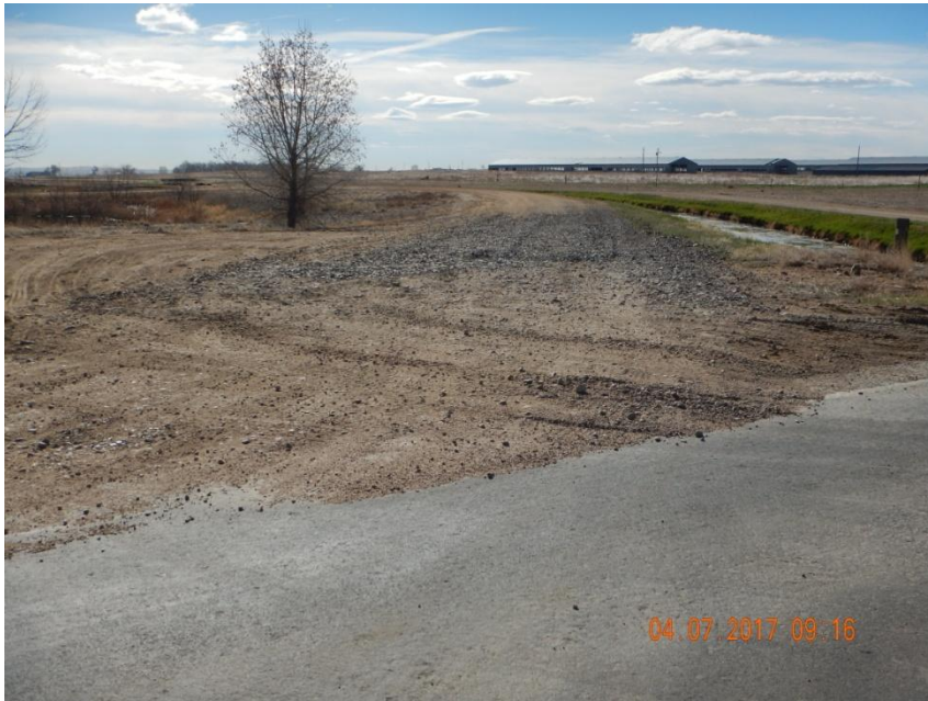
Photo 1. Photo taken from the entrance of location, facing East. Vehicle tracking pad installed but does not appear to be a sufficient amount of material. Monitor vehicle tracking and potential sediment discharge.
