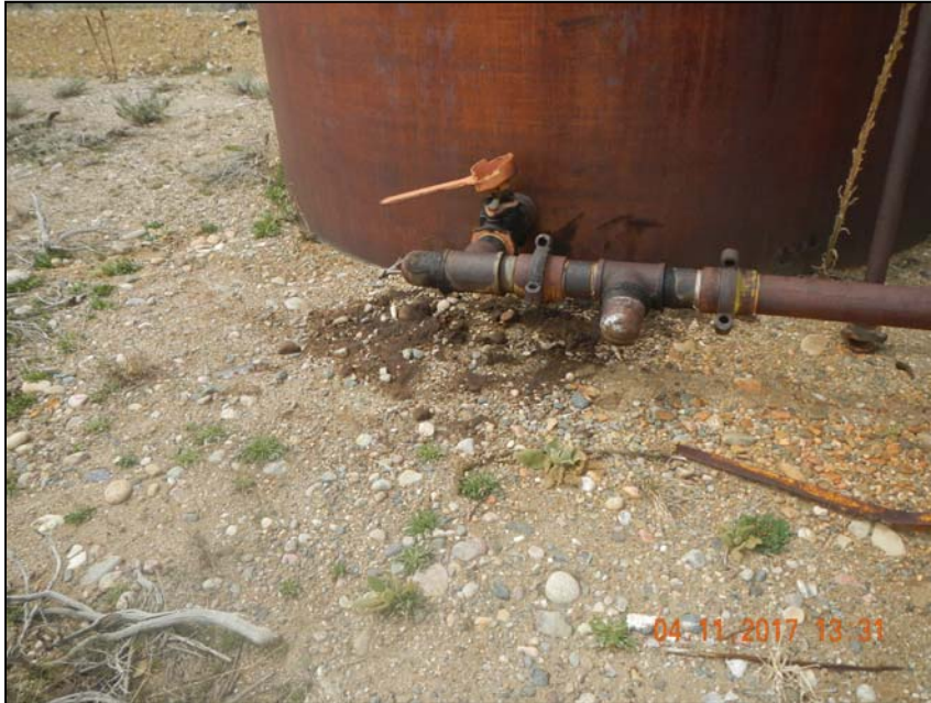
Photo 2. Stained soil at tank base of crude tank near wellhead.
