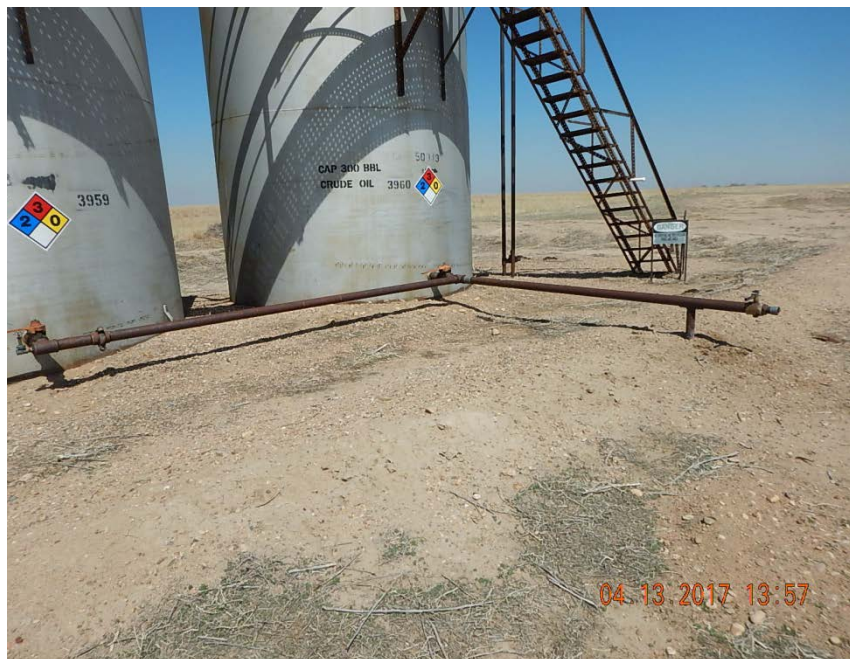
Photo 8: Low berms at tank battery
