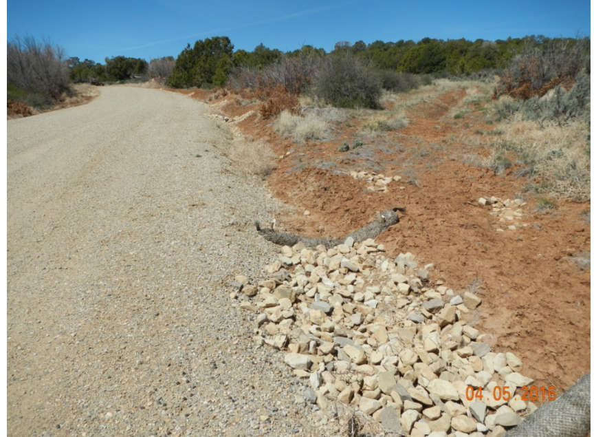
Photo 6: View of stormwater controls along the access road, appear to be functioning.
