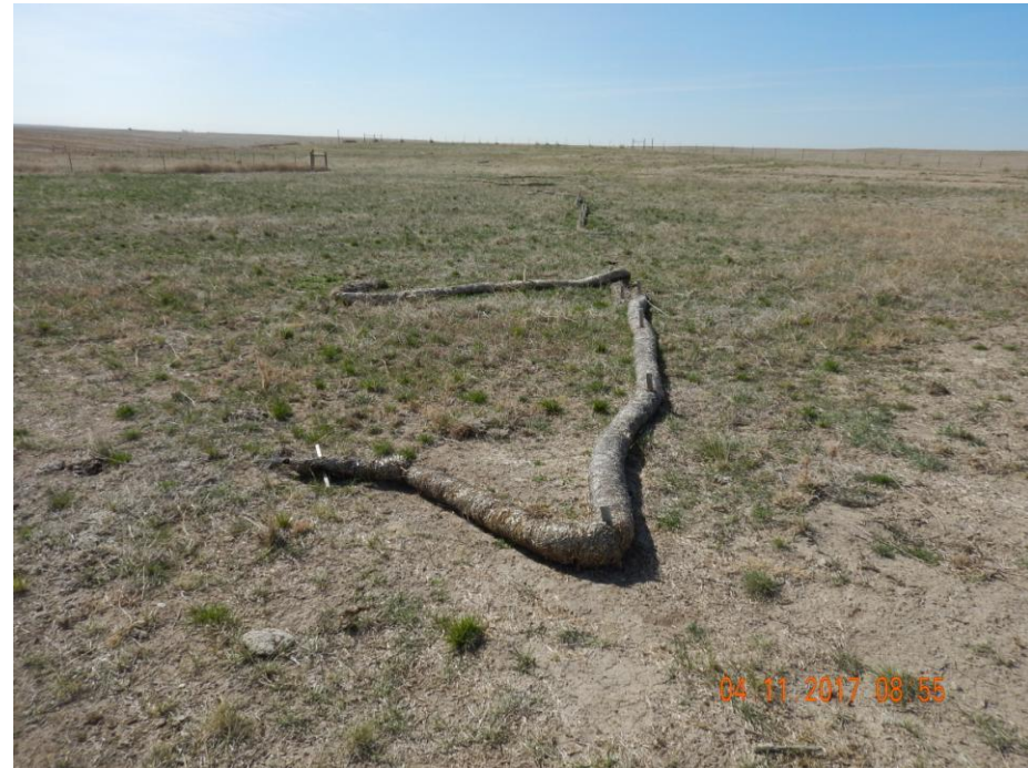
Photo 4: Photo taken from location. Photo shows straw wattles on the location have not been maintained and are in disrepair. Wattles in current condition is debris and needs to be either repaired or removed.
